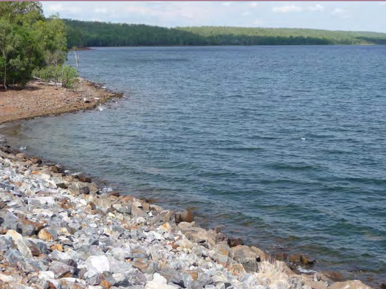
Darwin River Dam was constructed in 1972 and is designed to supply 200,000 people. Photo: John Drewry
