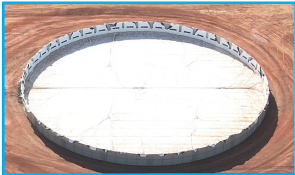
Typical Water Storage Tank
