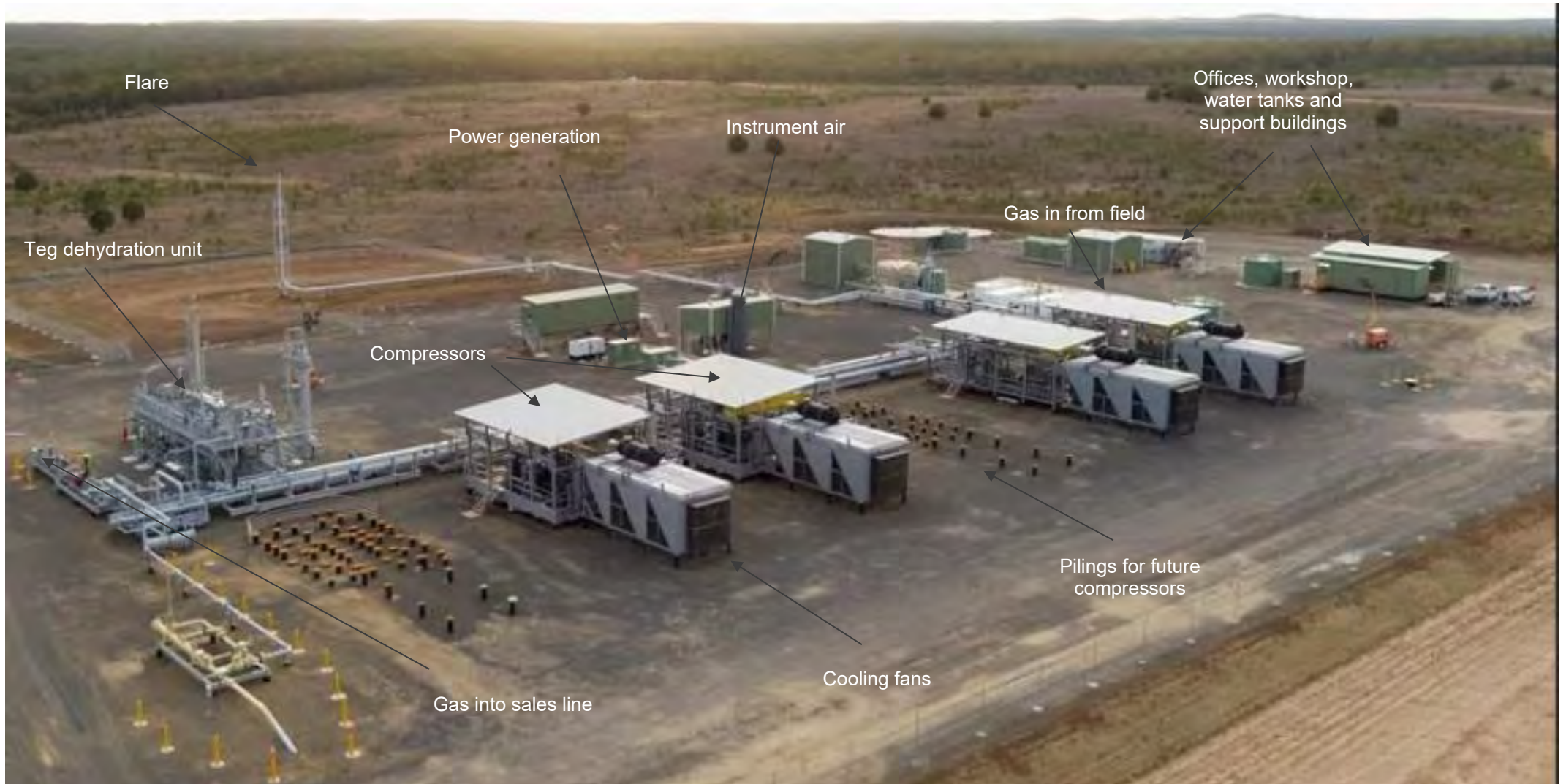
Figure 6 Analogue site for the Sturt Plateau Compression Facility (similar Senex Roma North Facility)
