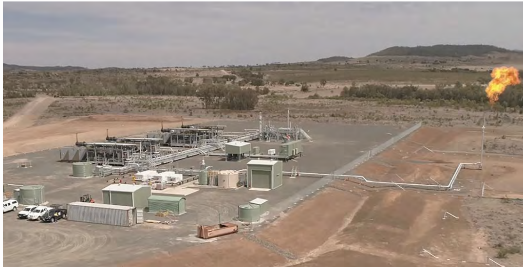
Example of compressor station (flare not routine)
