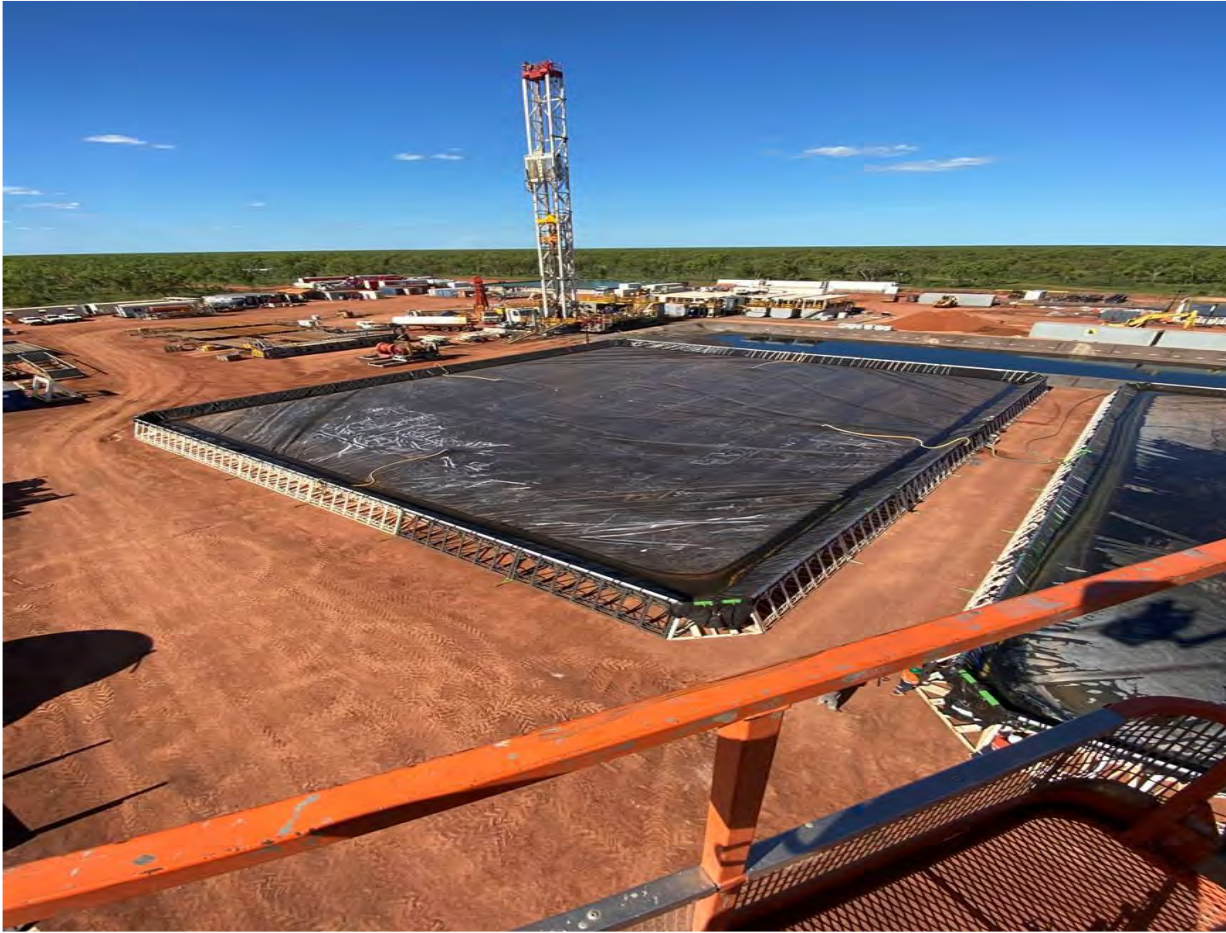
Figure 32: Example of covered water storage tank located on the existing Kyalla 117 N2 site
