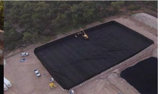
4. Geomembrane installation
