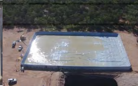
7. Secondary liner installation
