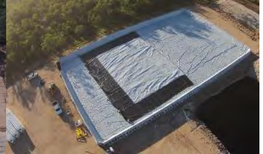
8. Primary liner installation
