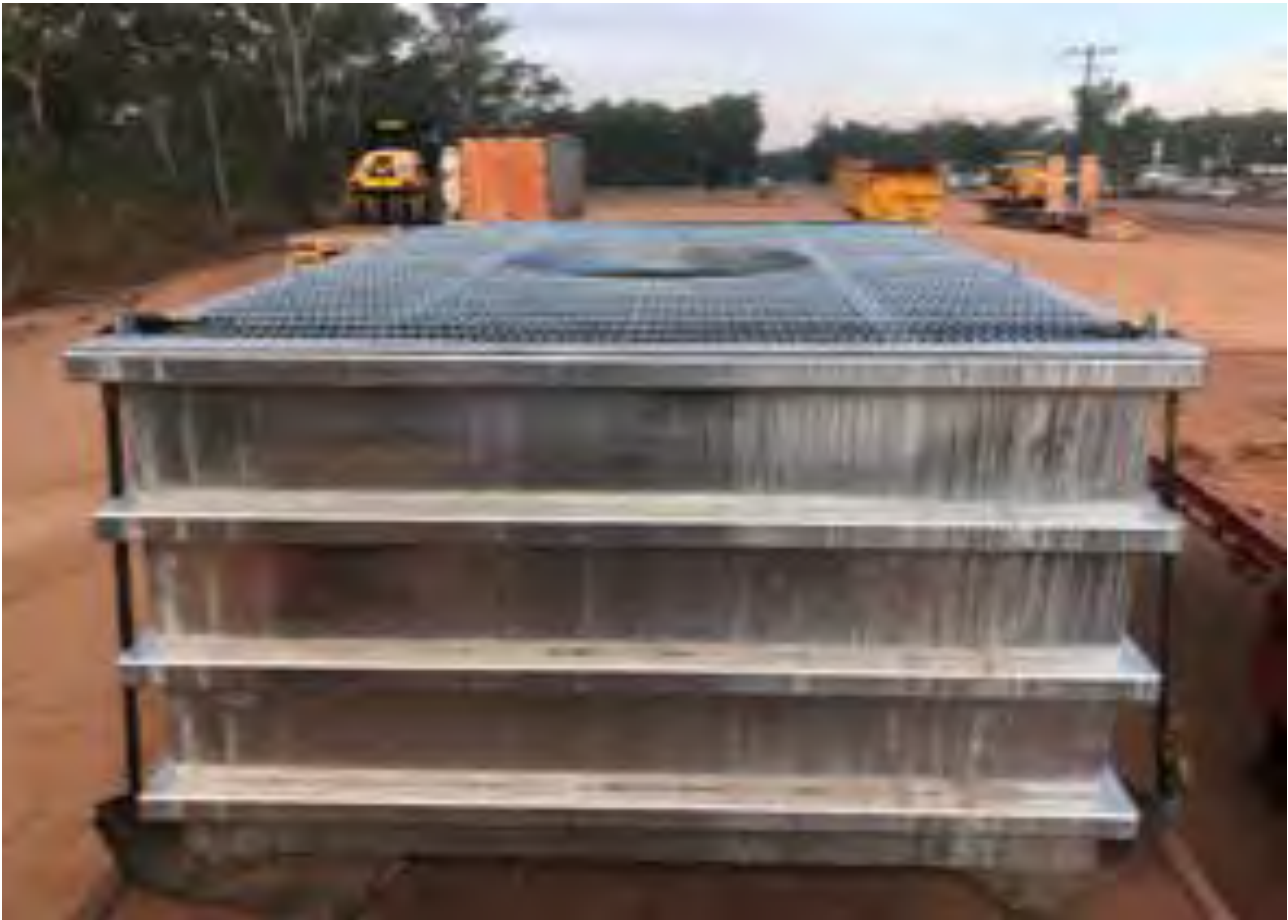
Figure 14: Picture of a cellar prior to installation
