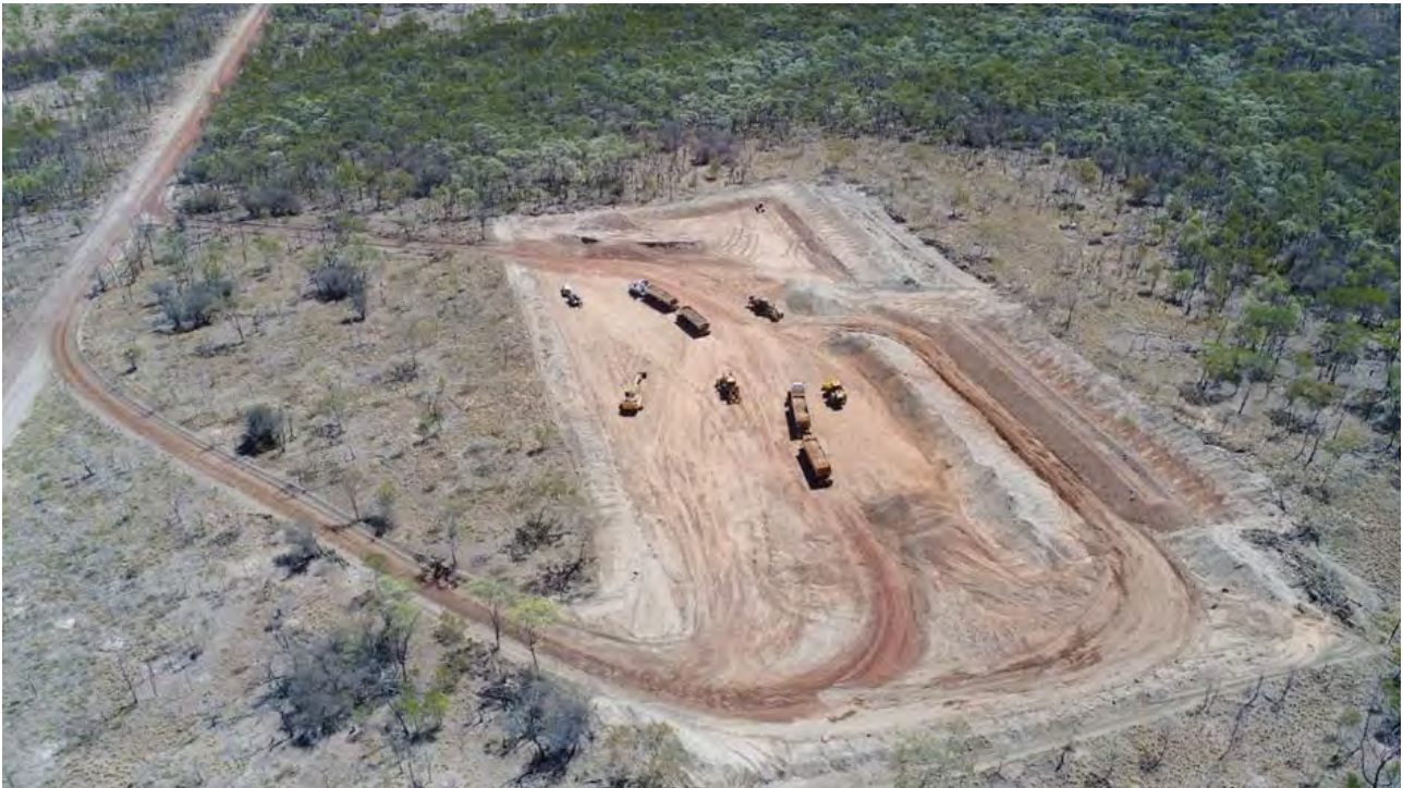
Figure 15: Example of a typical operational gravel pit
