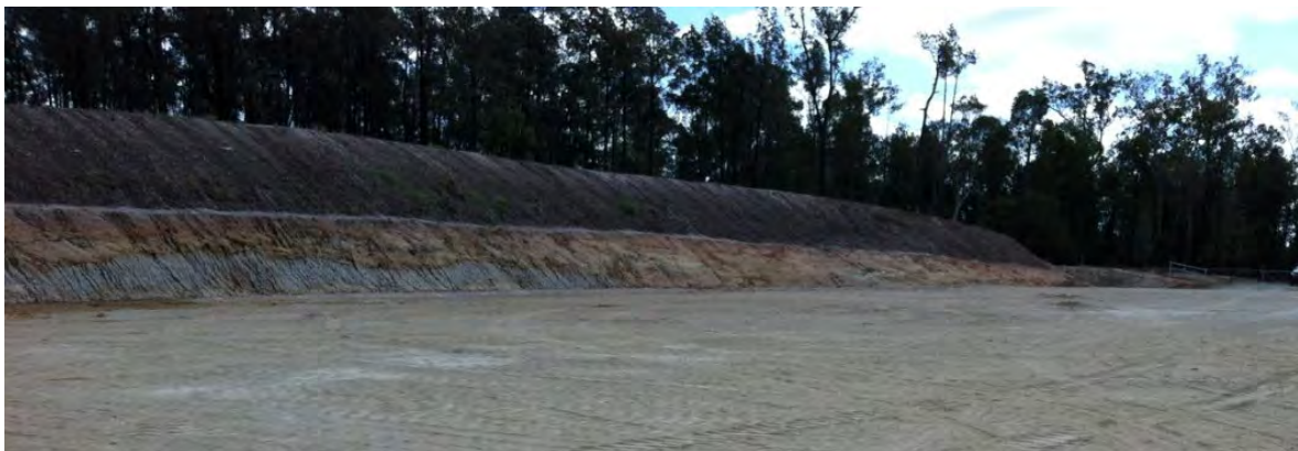
Figure 2.18: Topsoil windrow above the cut batter used to divert clean water away from the wellpad
