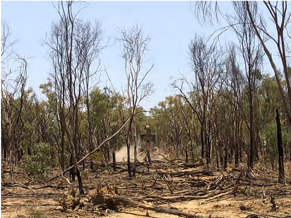
Figure 2.6: Respreading Acacia shirleyi over a seismic line during rehabilitation
