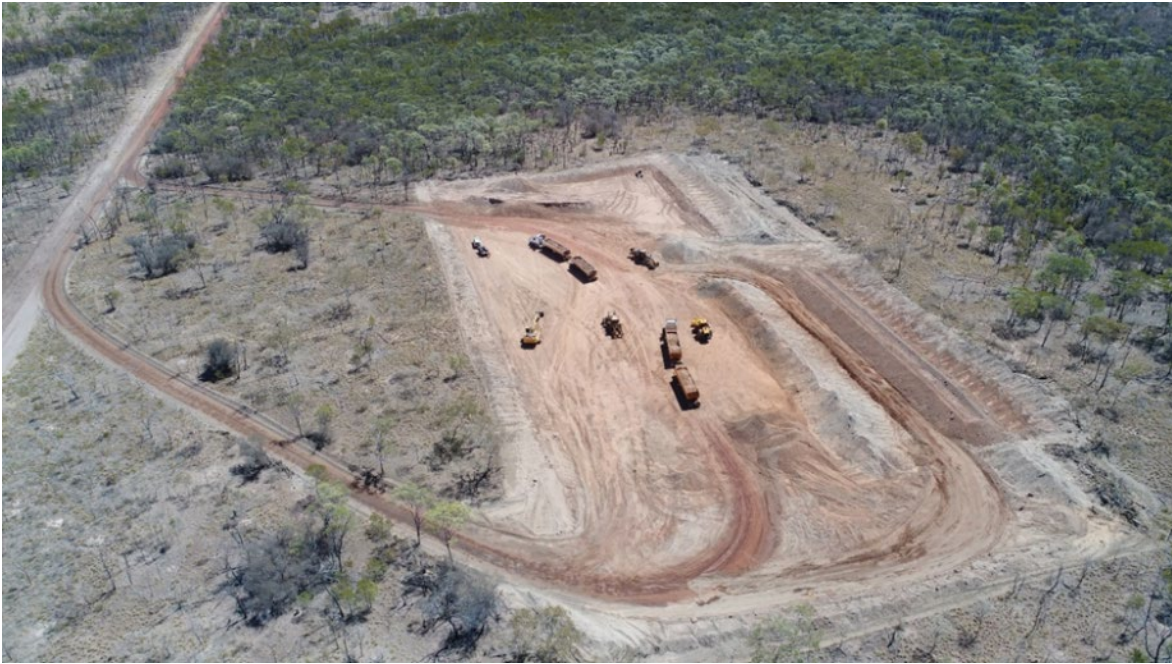
Figure 13: A typical operational gravel pit
