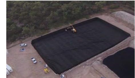
5. Geomembrane installation
