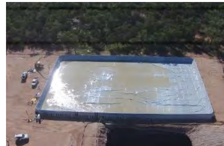
7. secondary liner installation
