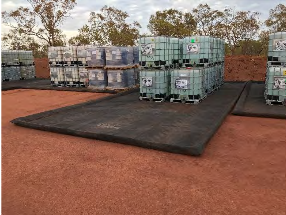
Figure 10: Example of spill mats used to contain drilling and tarps to protect sand.
