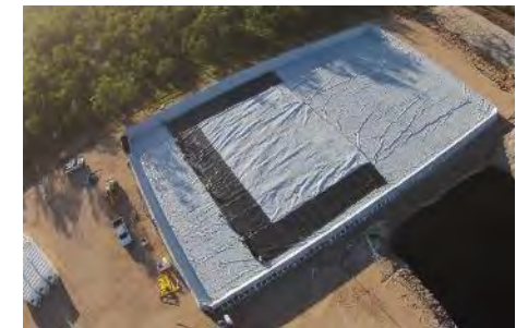
6. Primary liner installation
