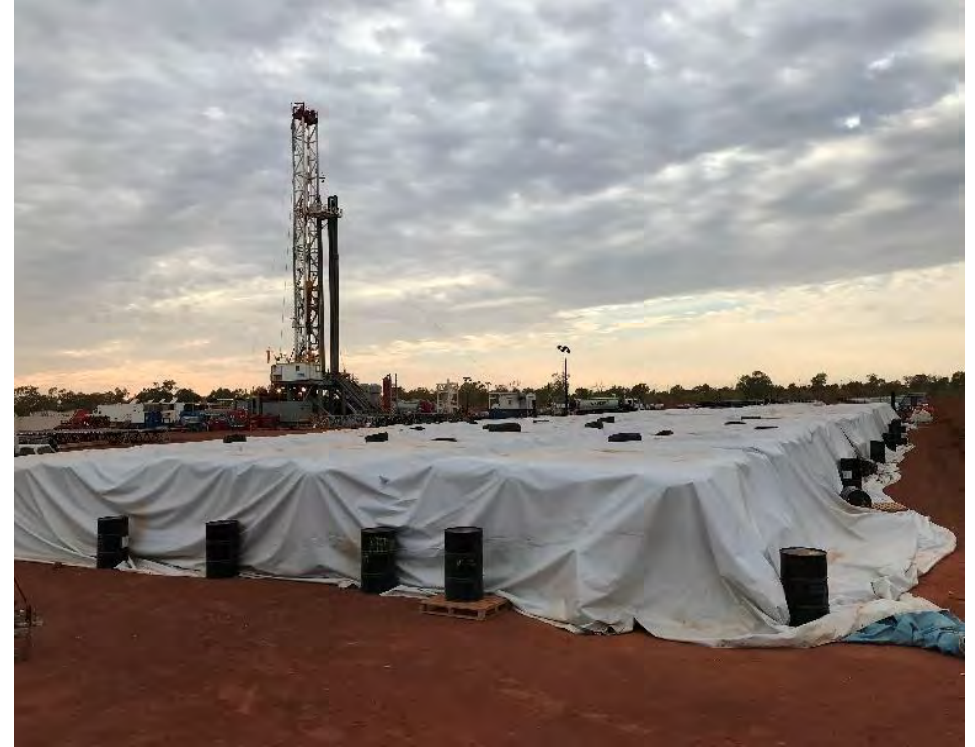
Figure 10: Example of spill mats used to contain drilling and tarps to protect sand.
