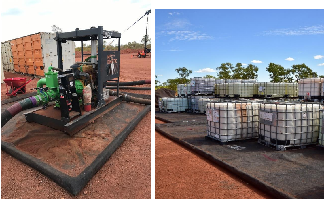
Figure 28: Example of spill mats used to contain stimulation additives and under a pressure pumping unit
