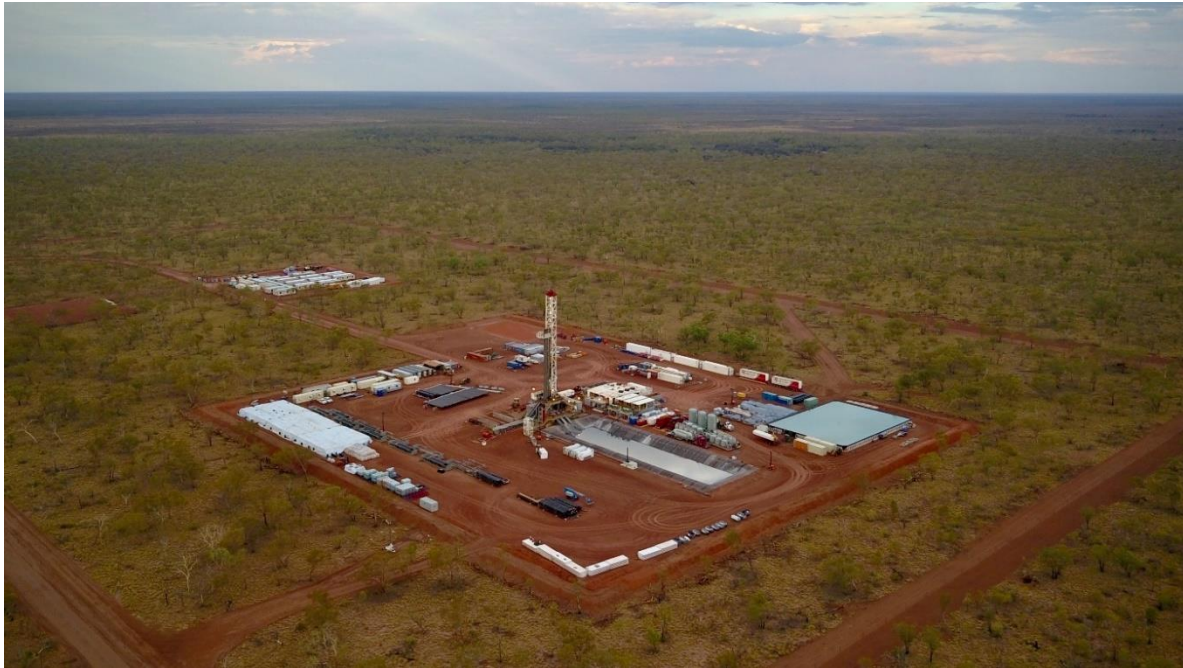
Figure 3: Existing Kyalla 117 N2 disturbance footprint including lease pad upon which the Kyalla 117 N2-2H and Kyalla 117 N2-3H wells and associated activities will be located (image taken during drilling of Kyalla 117 N2-1H)
