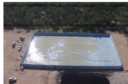
7. secondary liner installation
