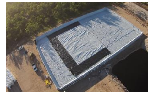
6. Primary liner installation
