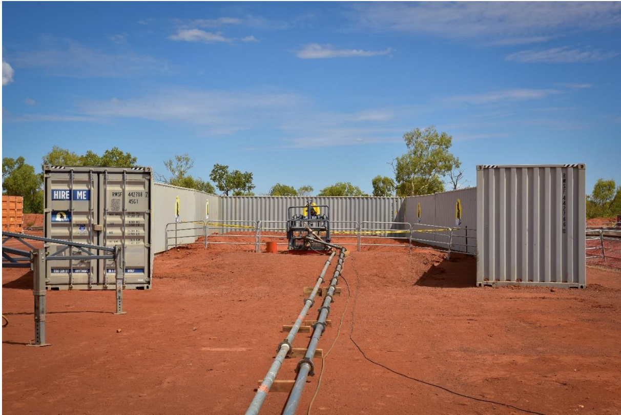
Figure 22: Horizontal flare set up (Note: the pit has a coletanche liner located ~500mm below the surface)
