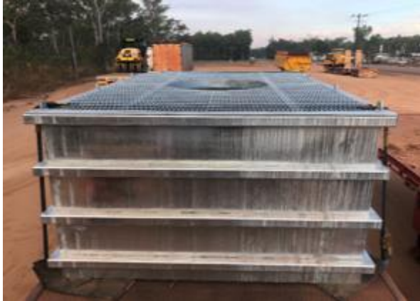
Figure 8: Picture of a cellar prior to installation
