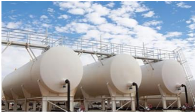
Figure 23: Example of condensate storage tanks (image provided for indicative purposes only)
