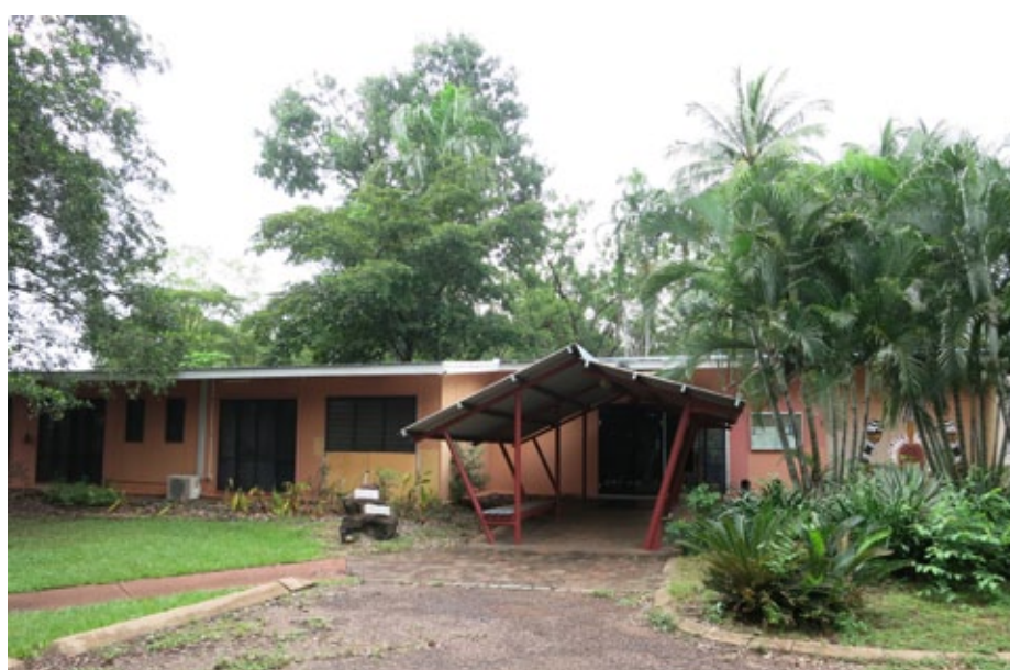
Old Batchelor Hospital
