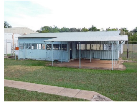
Fig.30 - South facade of the Ablutions block.
