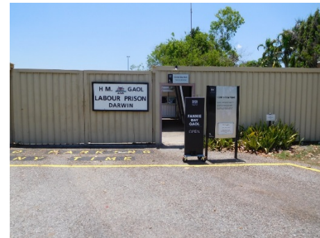
Fig.04 - Western facing perimeter wall showing the vehicle entrance gates and pedestrian entrance gate. The wall dates from ca 1976.
