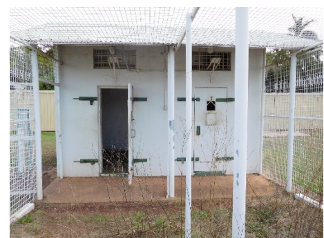
Fig.34 – cell doors from the exercise yard. Pedestal fans, directed into the cells, were fixed to the brackets seen in front of the two high level windows.
