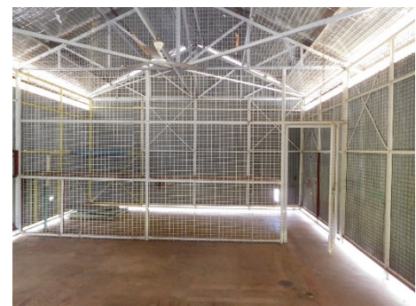
Fig.23 - Interior looking south. Note the weldmesh internal partition forming a cell.
