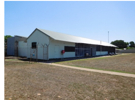
Fig.42 - South and west facade of the Kitchen and mess.
