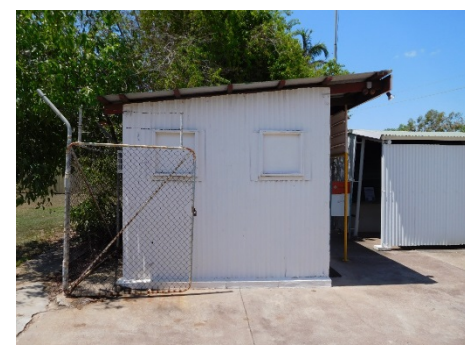
Fig.17 - North façade of the Reception building.
