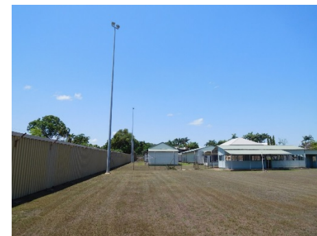
Fig.05 - Eastern perimeter wall looking south from inside the gaol.
