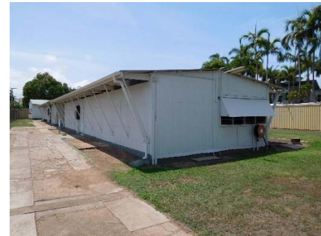
Fig.45 - North and west façade of the Stores building.
