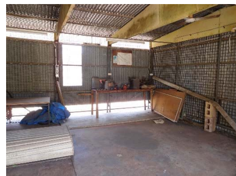
Fig.49 - Interior of the workshop in the eastern side of the building.
