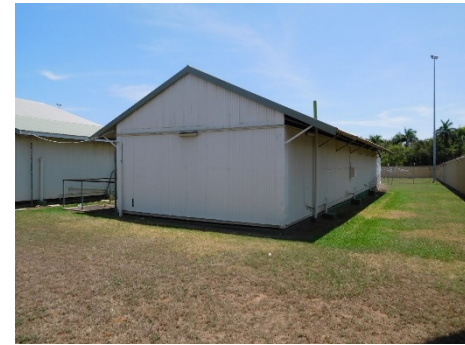
Fig.22 - South and East façade of Cell block D. Cell block C is to the left and the perimeter wall is to the right.
