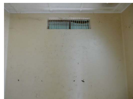
Fig.61 - Interior of the cell looking at high level barred windows located in the end walls (east and west facing).
