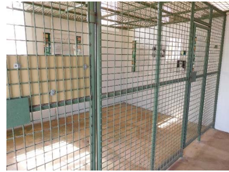
Fig.55 – Cell area with open weld-mesh cells.
