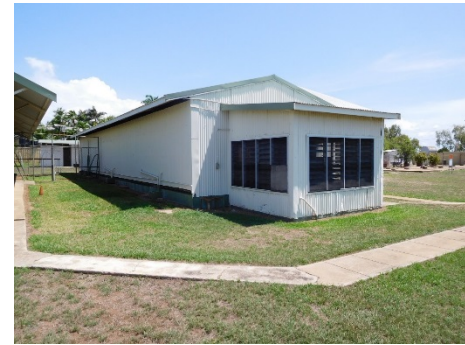
Fig.25 - North and east façade of Cell block C. The annexe for the senior guard is on the northern end of the cell block.
