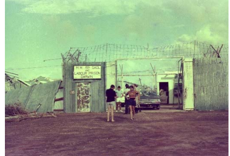
The entrance to HM Gaol, East Point Road after cyclone Tracy, ca 1975.
