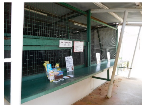
Fig.12 - Non-contact visitor's area – currently the access walkway from the main gate.
