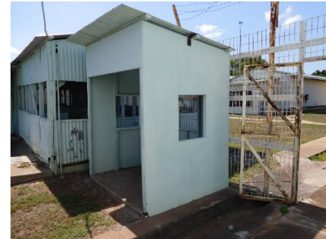
Fig.28 - View of the Guard house. The Ablutions block is immediately adjacent.
