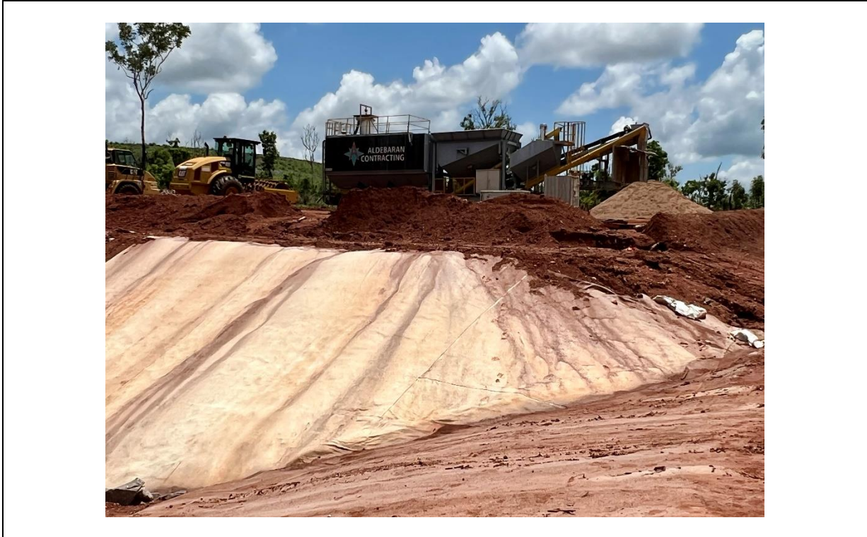
Plate 5 Matting geotextile for culvert crossing works (erosion and sediment control)
