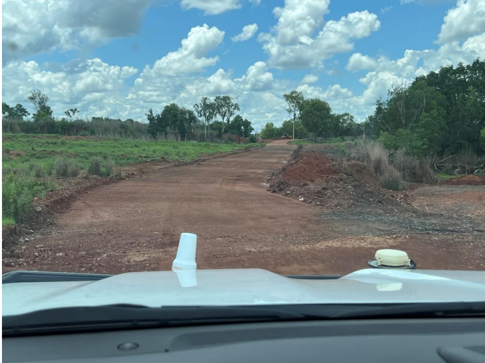
Plate 3 Internal road upgrade works as part of PRAP
