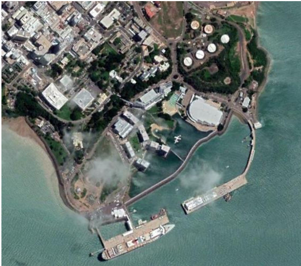
Figure 4: Aerial image of the locality
