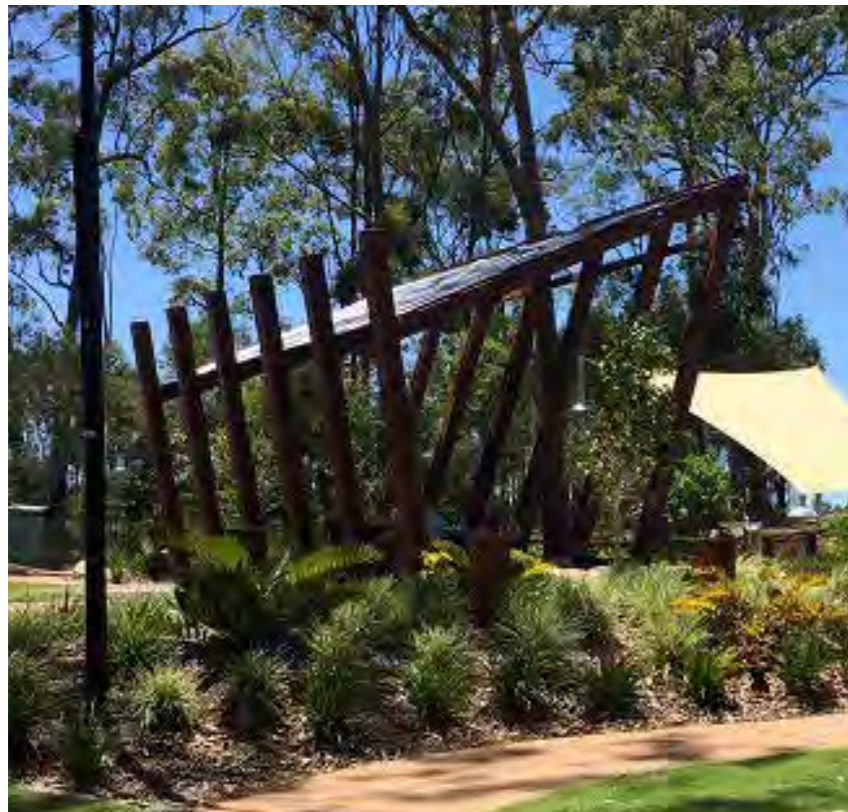
Nest-like shade structure nestled within shade trees and planting, providing passive cooling.
