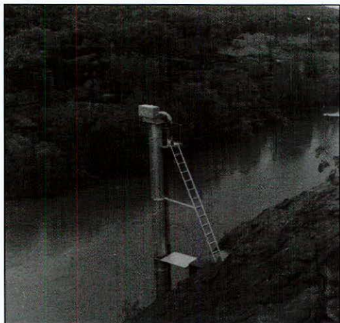
A recorder tower at South Alligator River
