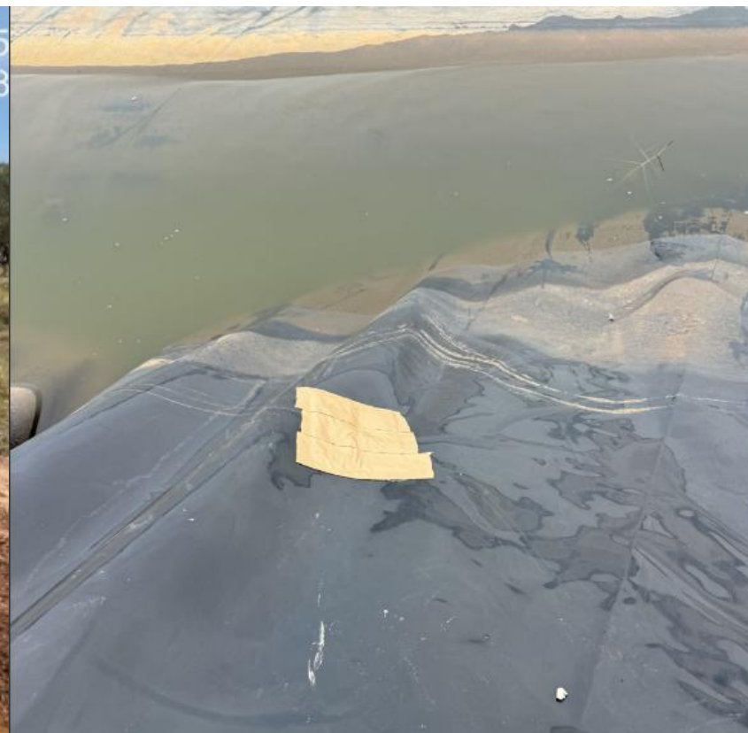
Cause of Affected Rainwater on Mandatory Tank Cover (tear now covered by patch)
