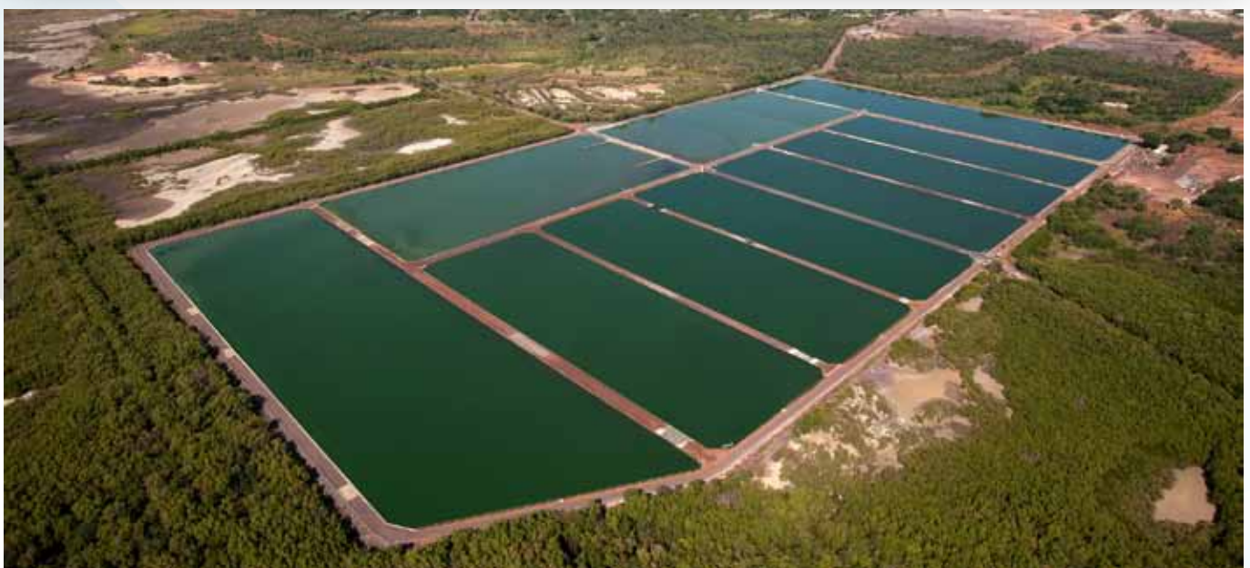
Leanyer – Sanderson wastewater treatment plant. Sewage is treated biologically as it passes through a series of lagoons, and then released to Buffalo Creek in Darwin Harbour.
