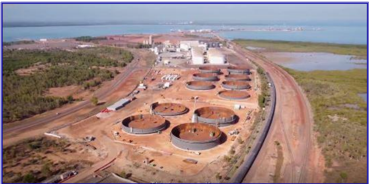
Figure 1-1 Crowley BFSF under construction at East Arm Wharf (Crowley)
