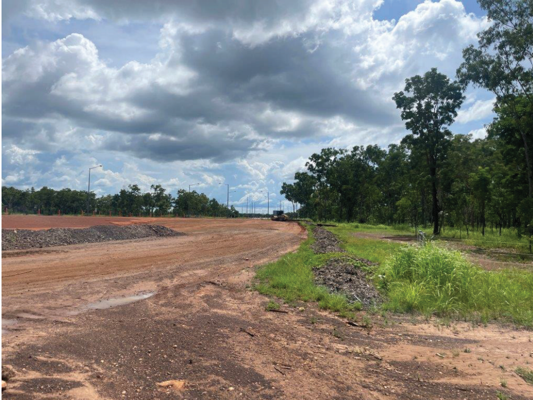
Gap in Mulch Berm for access track. To be closed off with a trafficable berm.
