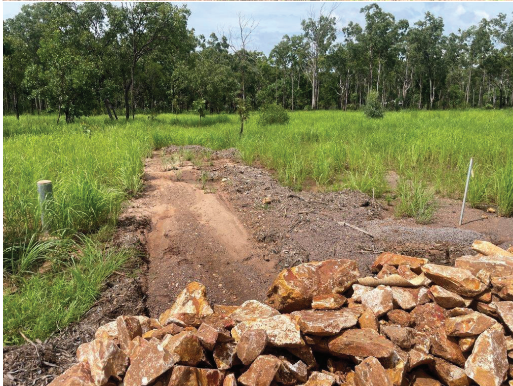
Evidence of Sediment Deposition past breached sections of mulch berm. Sediment to be cleaned up so far as reasonably practicable.
