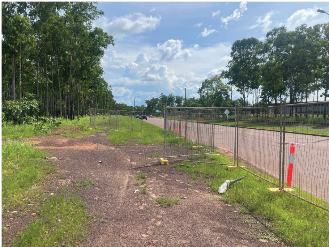
Sediment wash off onto PRH Access Road 2 from existing power track (appears historical)
