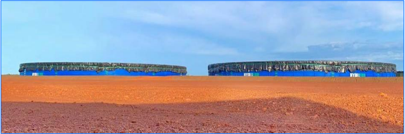
Figure 23: Example of above ground water storage tanks
