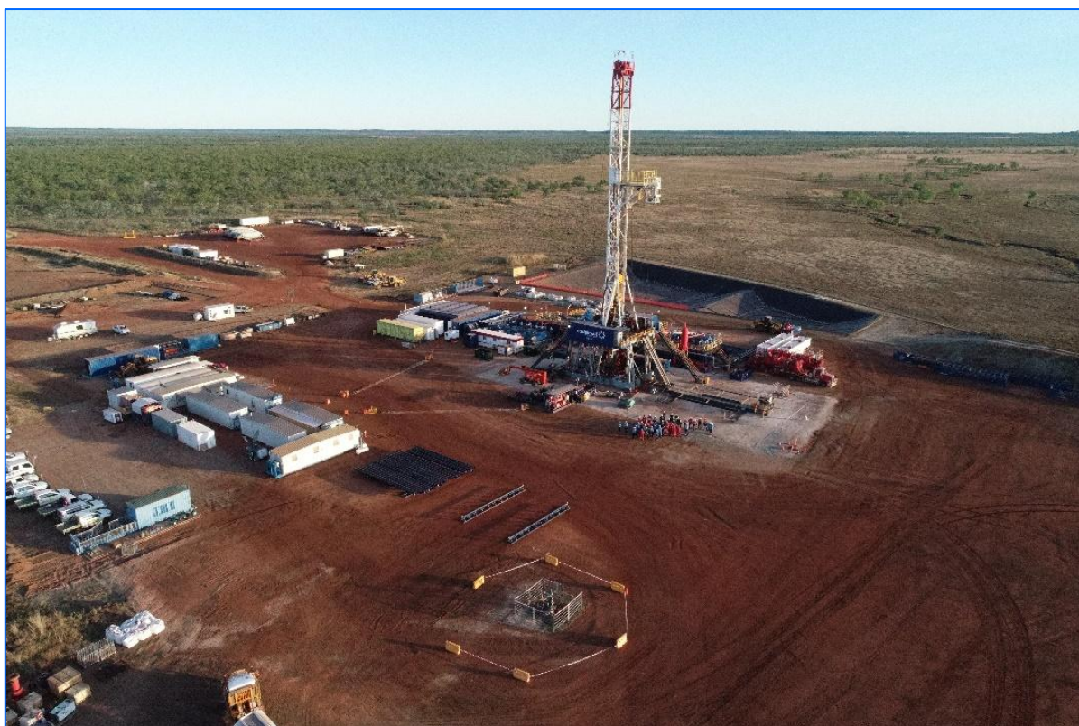
Figure 8: Mount Brown well pad during drilling operations
