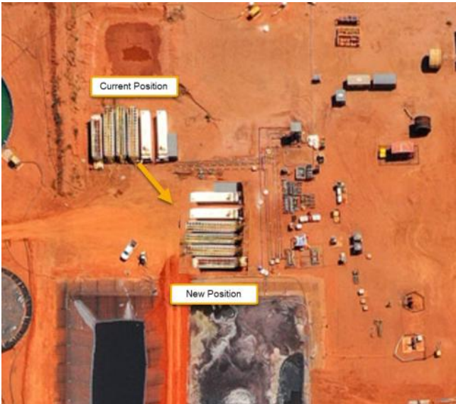
Planned tank move.jpg
