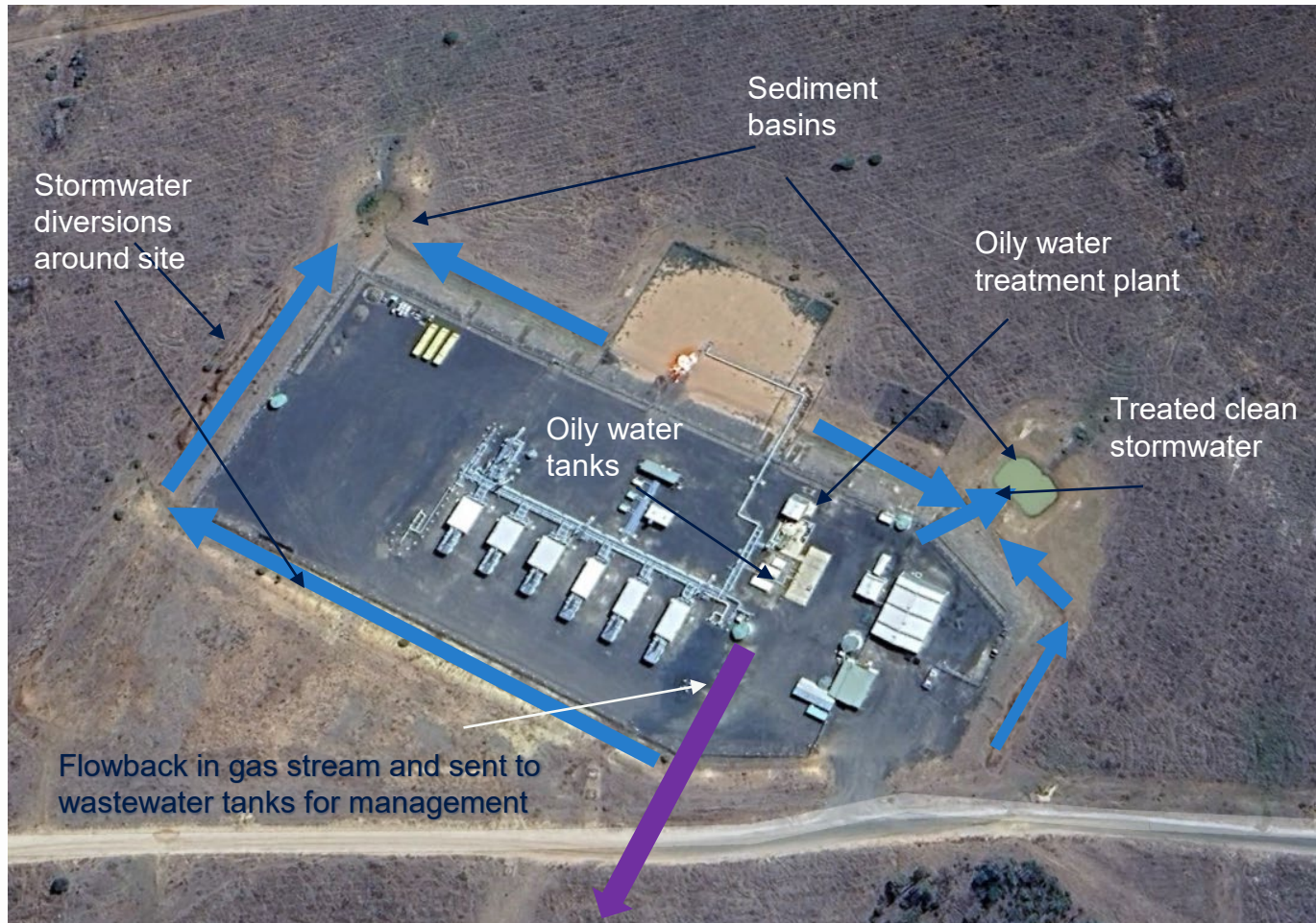
Aerial view of Jemena's Roma North gas compression facility in QLD
