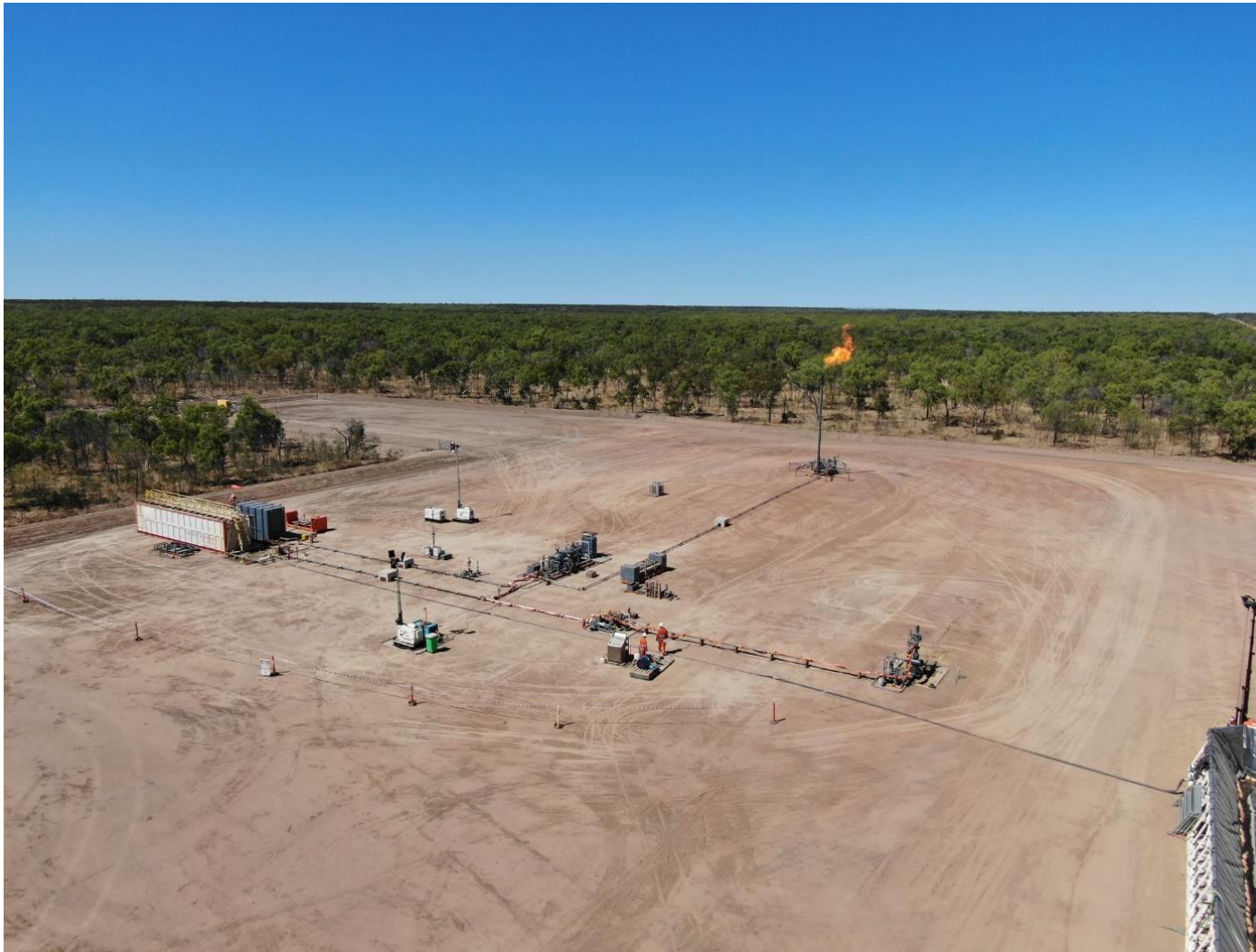
Figure 8 Example of a well test underway at the existing Amungee NW location – noting flaring will be minimal if gas is sold instead of flare
