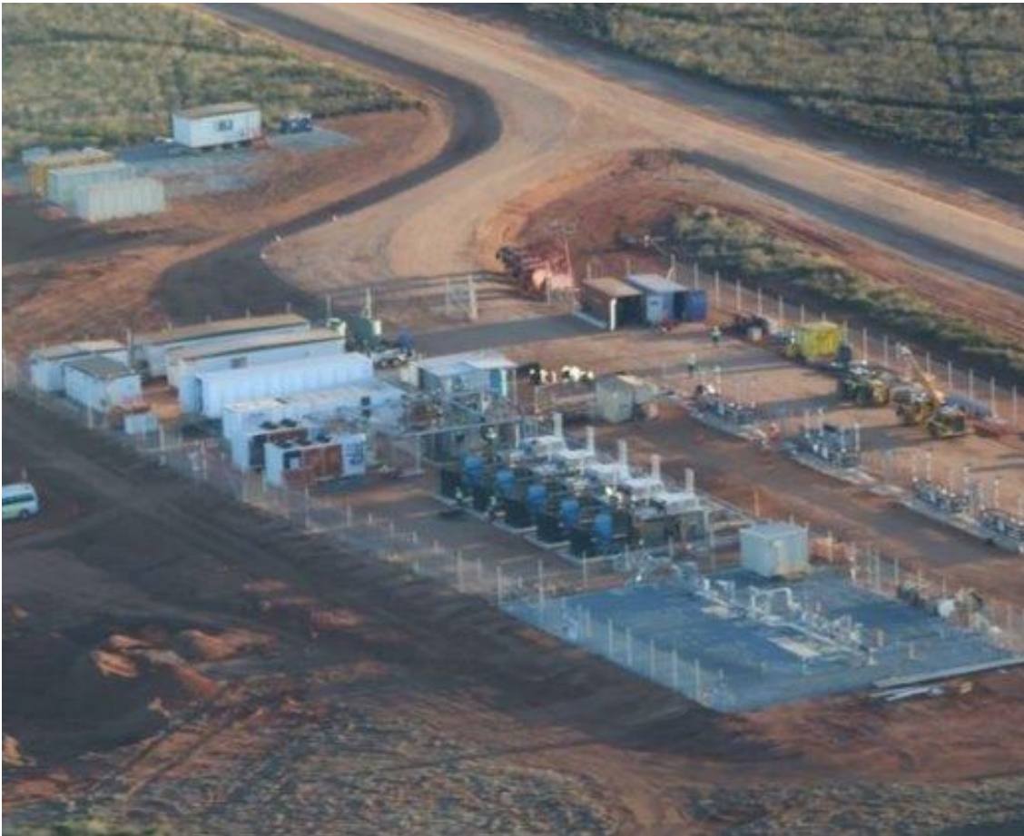
Figure 9 Example of a temporary gas processing facility used to compress and sell gas into the domestic gas market
