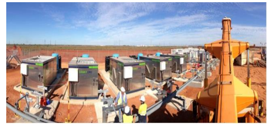
Figure 9 Example of a temporary gas processing facility used to compress and sell gas into the domestic gas market
