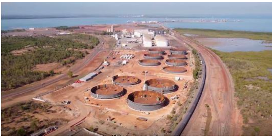
Figure 1 Crowley BFSF under construction at East Arm Wharf (Crowley)
