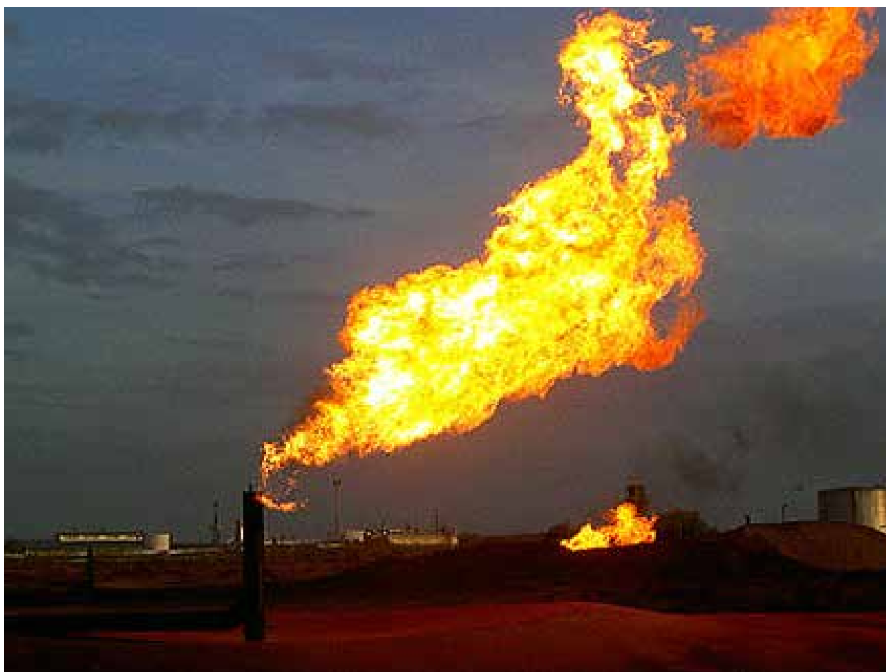
Figure 3. Natural gas flaring
