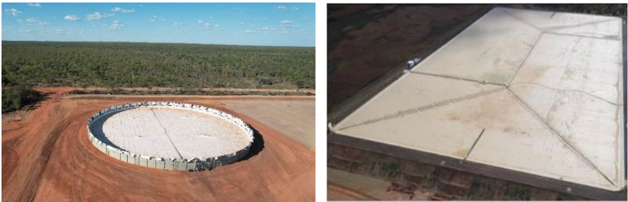
Figure 25: Examples of covered wastewater tanks used across Tamboran's sites (Riptide left; Flexipond right)
