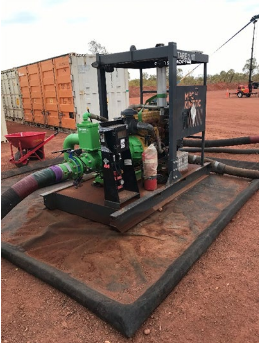
Figure 59: Examples of spill mats used to contain potential wastewater transfer spills
