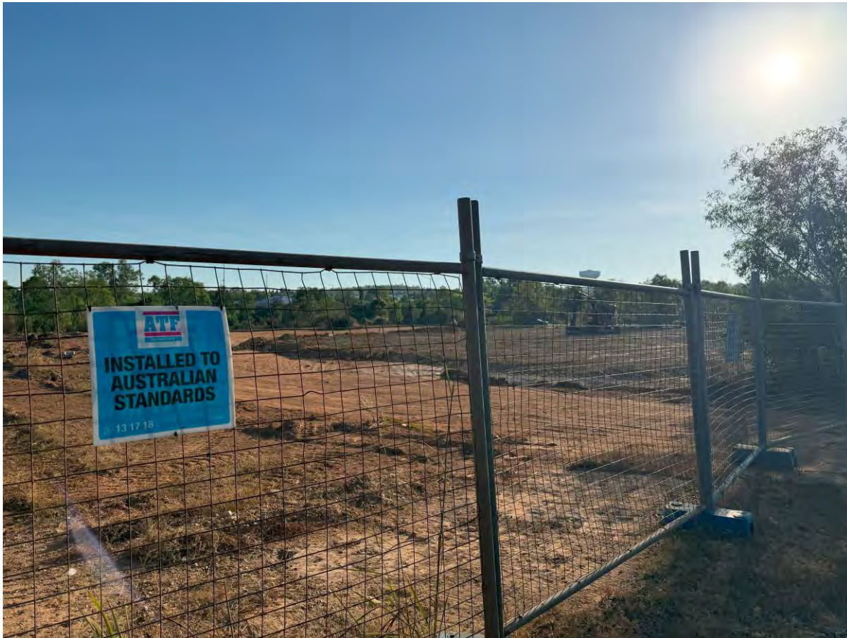
July 2026 photo of site – levels of site have been altered / not shown on drawings
