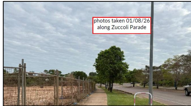
After clearing / earthworks commenced
