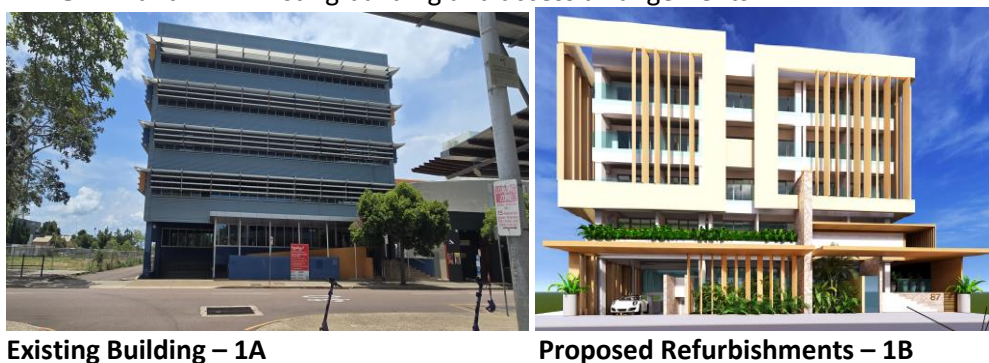
IMAGE 1A and 1B – Existing building and access arrangements
