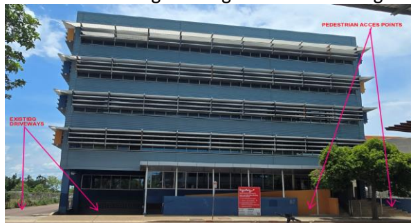
IMAGE 2 – Existing building and access arrangements
