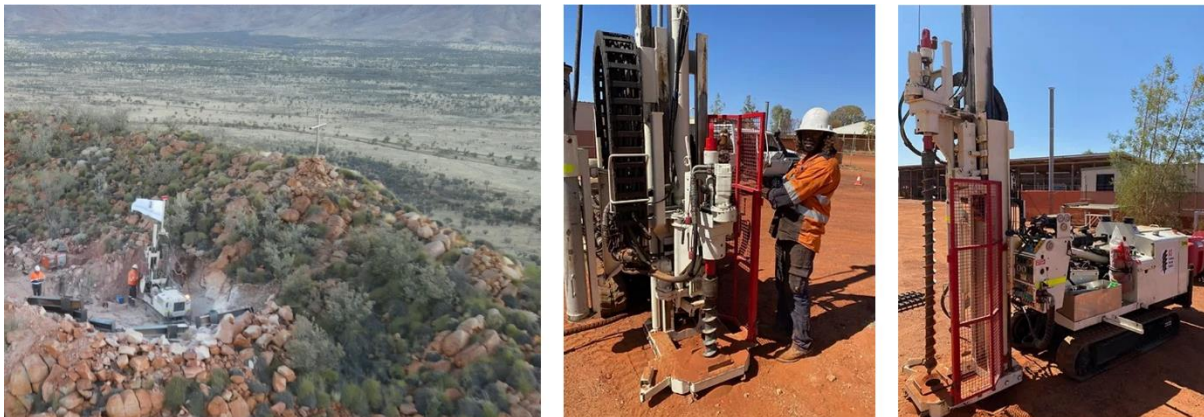
Figure 8: Small Geotechnical Drill Rig
