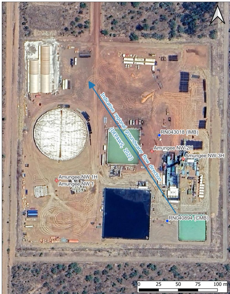
Figure 1 Site layout and indicative groundwater flow direction
