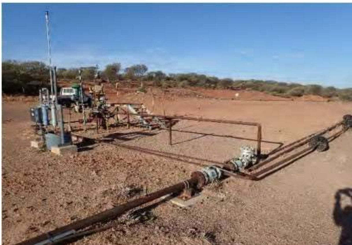
Figure 22: Typical well site layout and above-ground flowline
