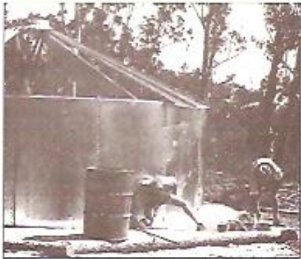
Installing a 10,000 gallon water tank at Bathurst Island
