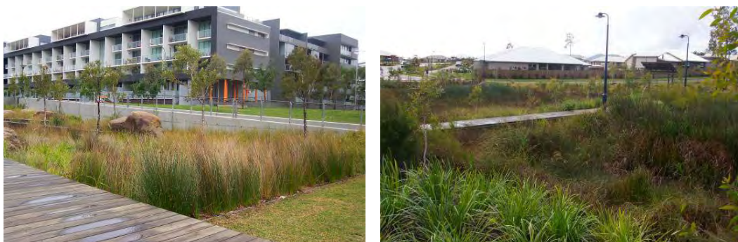
Figure 8.2: Examples of Bioretention systems to be used within the Bellamack subdivision to reduce loads entering nearby waterways.
