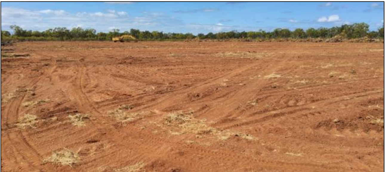
Figure 1: Typical conditions in the central part of the site at time of the investigation, looking southeast. Excavator is positioned at test pit TP02.
