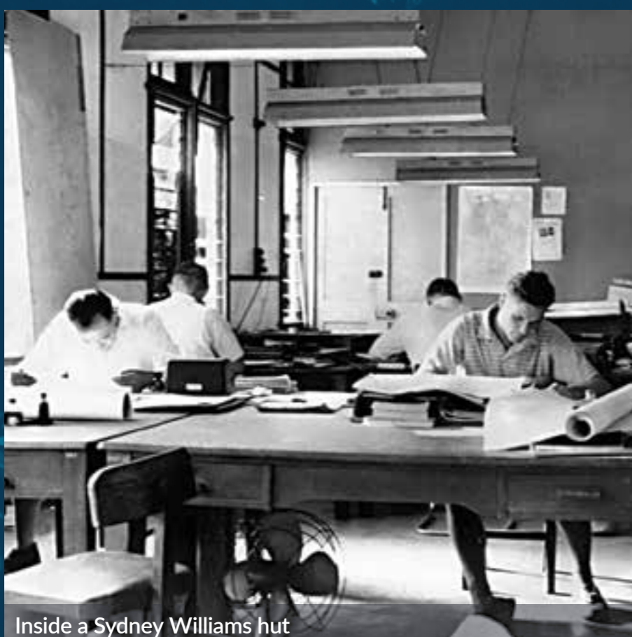
Inside a Sydney Williams hut
