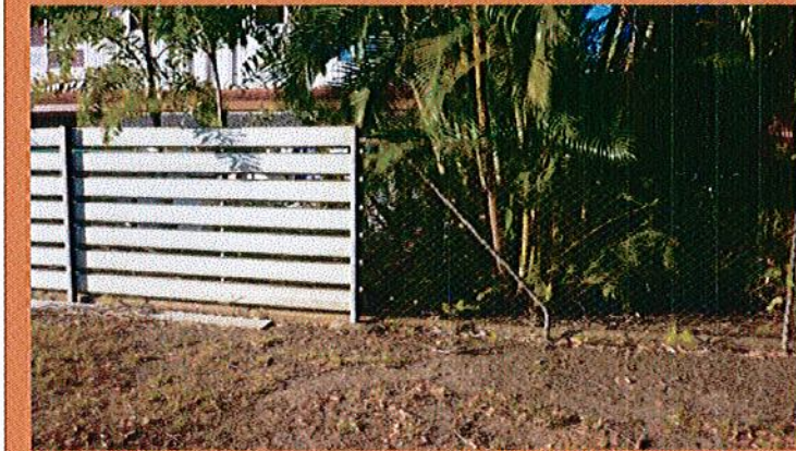
1800mm high metal horizontal cladding fence - southern boundary
