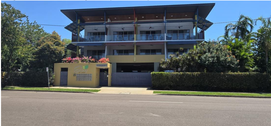
Image 2: The look of existing development, Parap Road view
