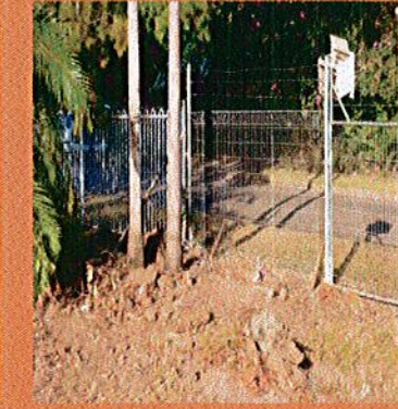
1800mm high Weld mesh fence north west corner
