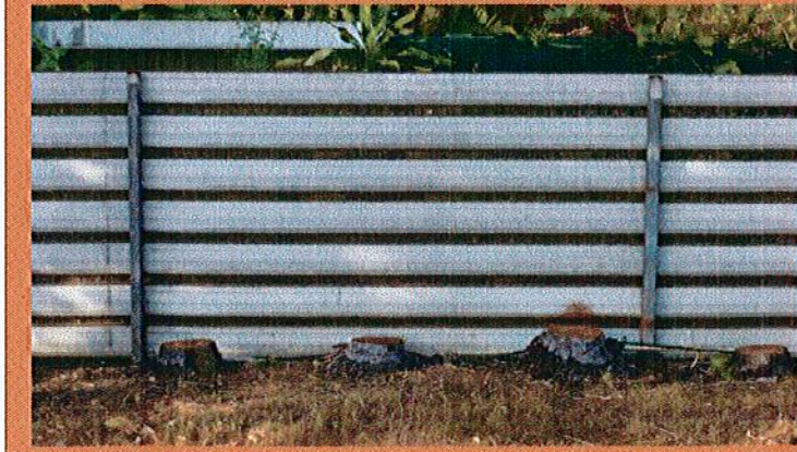
1800mm high horizontal cladding fence - southern boundary
