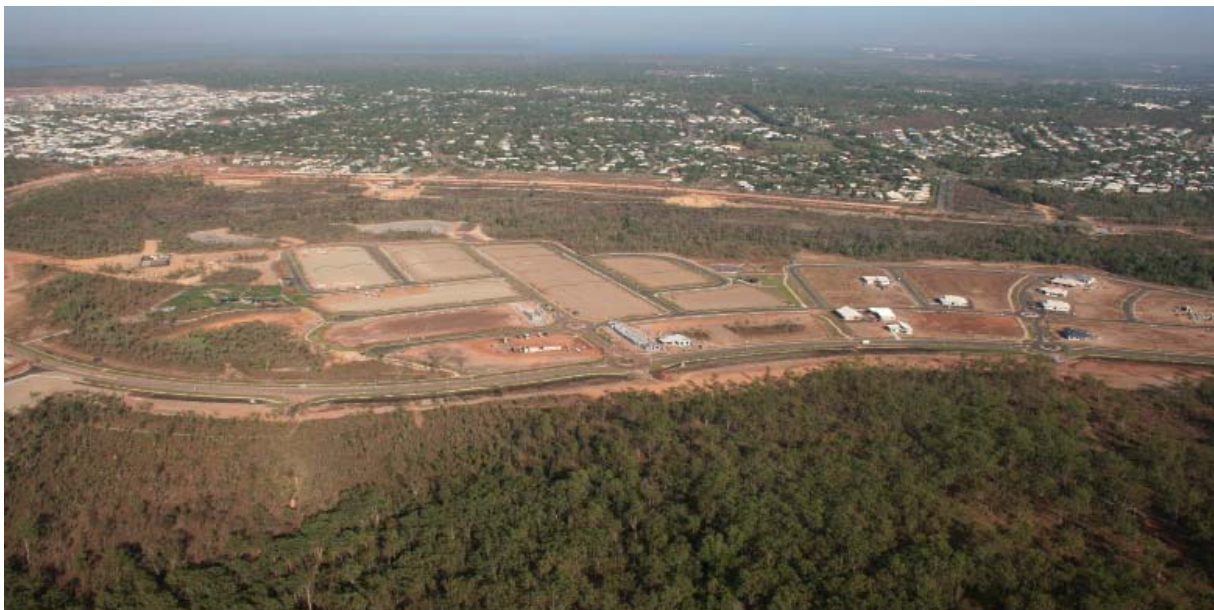
Johnston subdivision and WSUD treatments at the development stage. Photo: Phill Piper.
