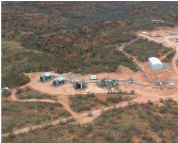
Figure 7: PVGF Central processing facility
