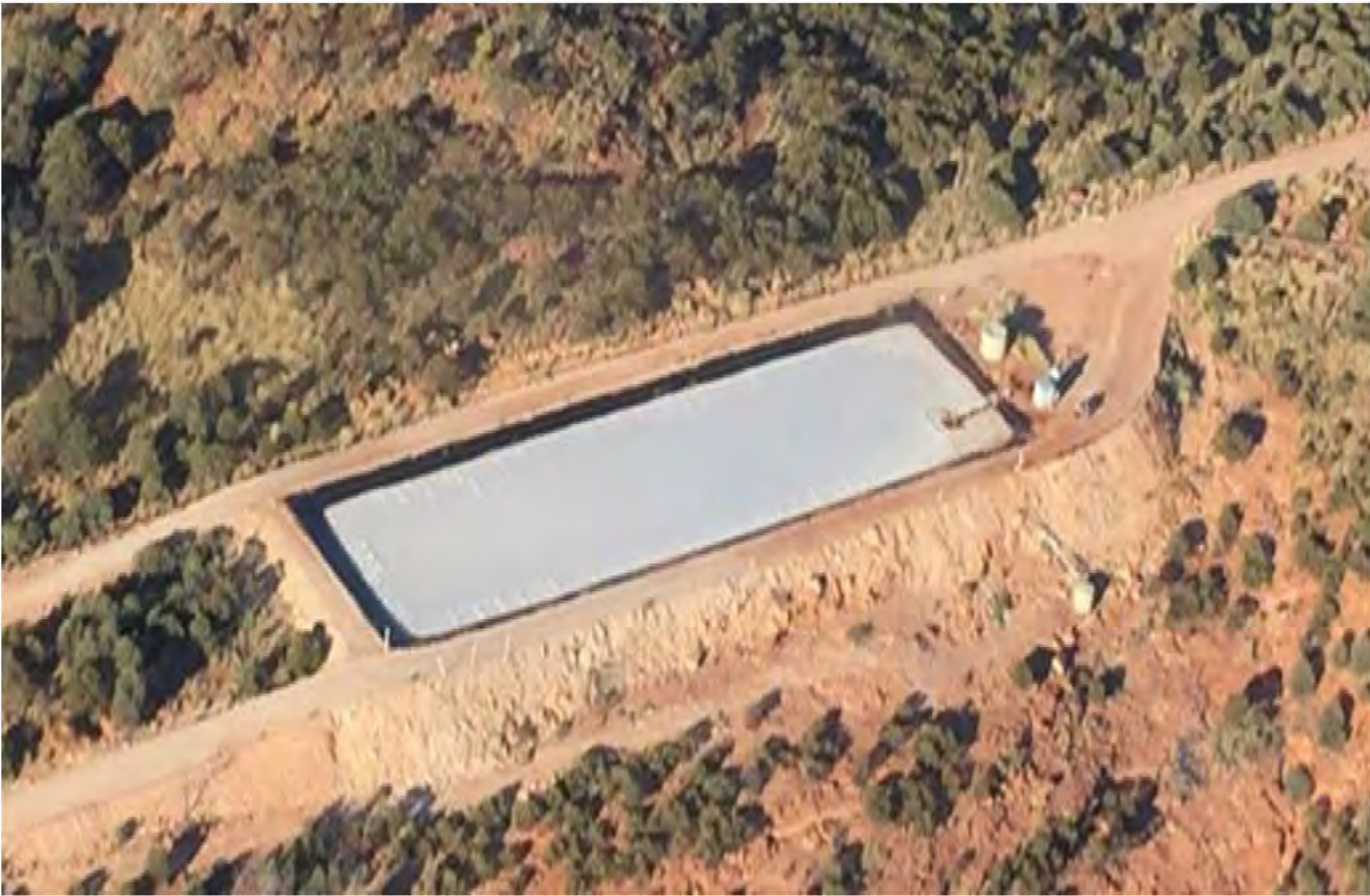
PV-09 evaporation pond
