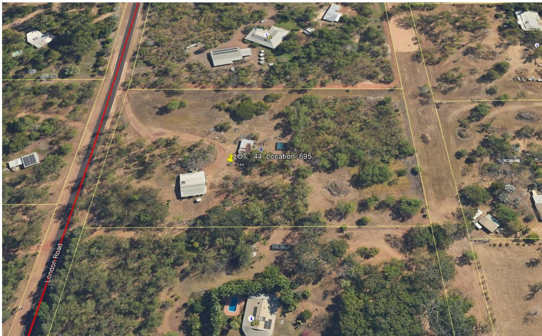
Figure 1 Subject site Lot 00044 Hundred of Strangways -65 London Road Virginia
