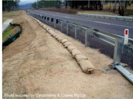
Photo 3 – Flow diversion berm used to minimise road runoff flowing down a steep, unstable section of the embankment
