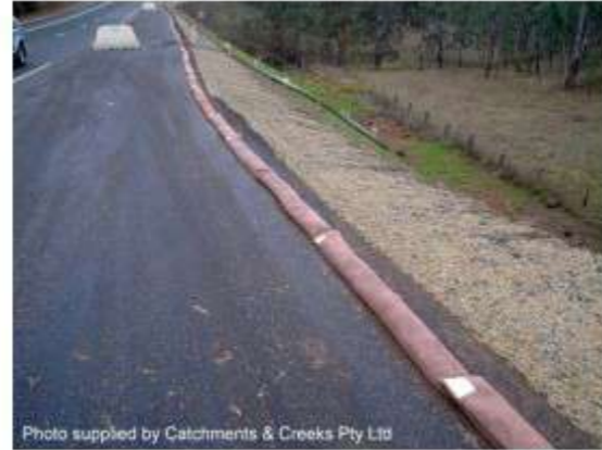
Photo 4 – Sandbag flow diversion berm used to minimise surface flow over a recently seeded embankment
