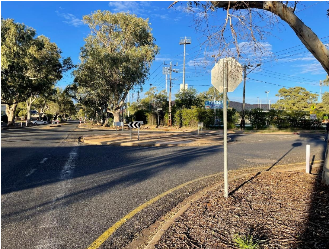
Figure A 28 Line marking in poor condition
