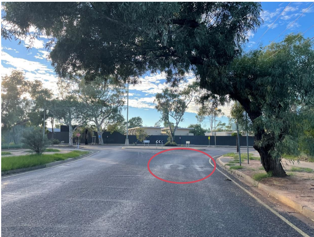
Figure A 6 Faded 40km/h speed limit pavement marking
