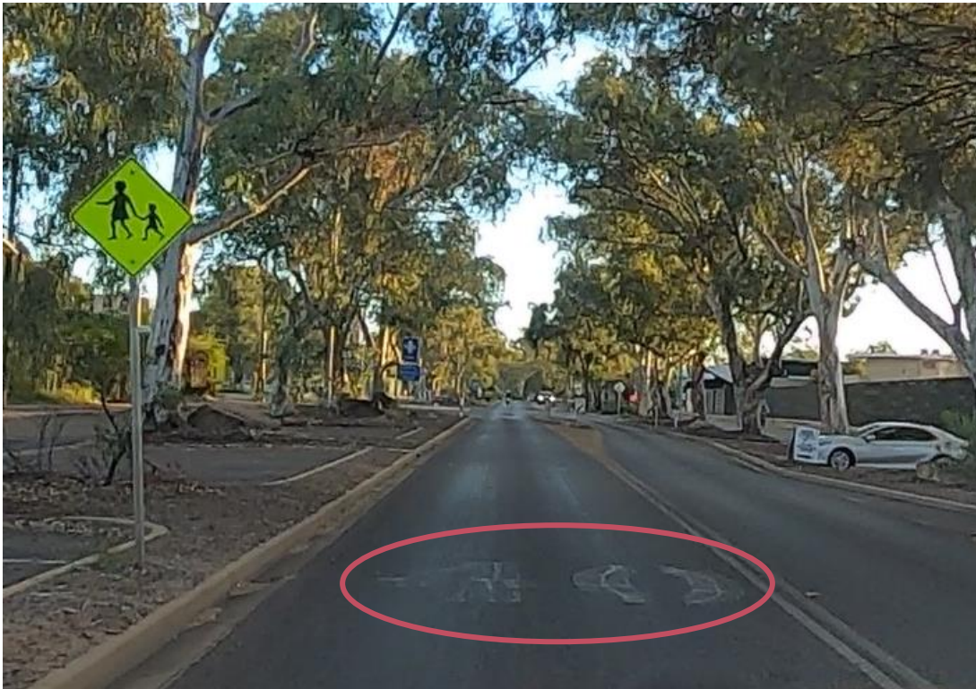
Figure A 8 Faded 40km/h speed limit pavement marking
