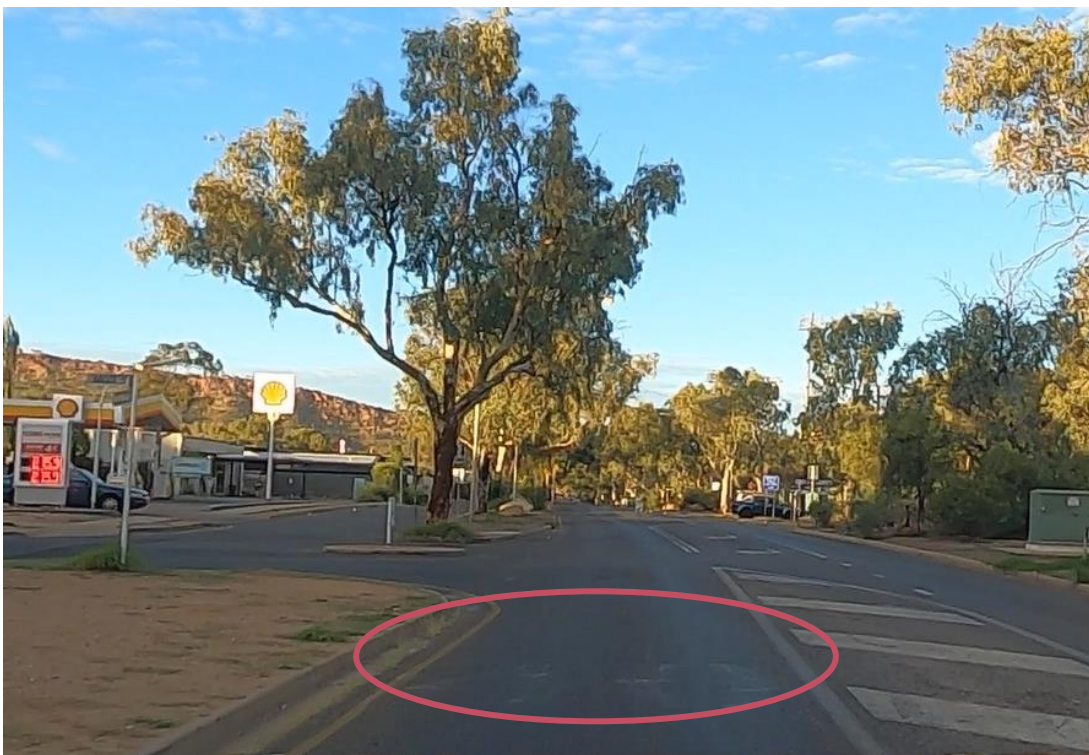
Figure A 8 Faded 40km/h speed limit pavement marking
