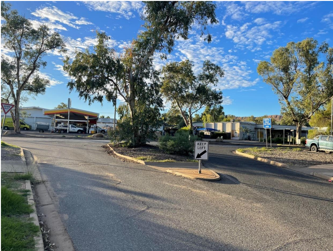
Figure A 26 Line marking in poor condition
