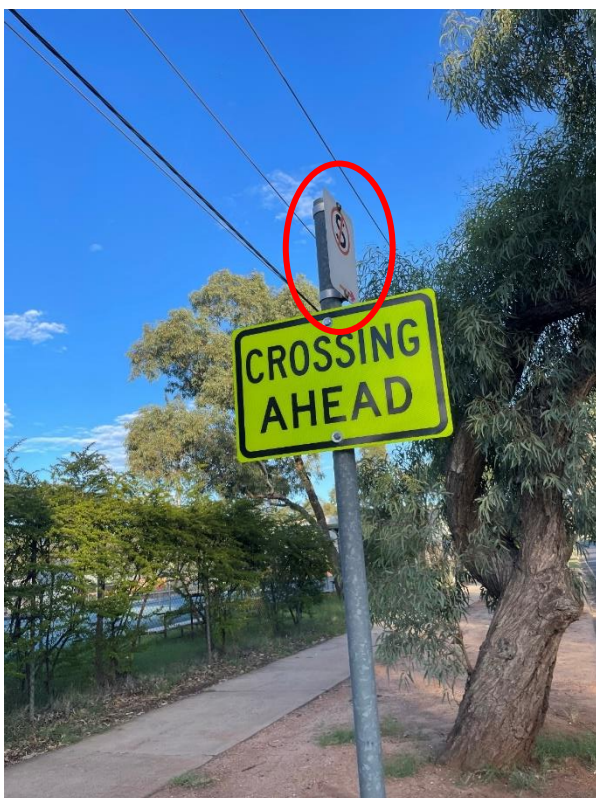
Figure A 12 Non-compliant 'No Stopping' signs
