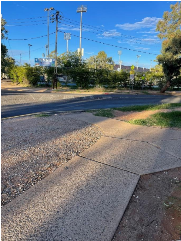
Figure A 10 Misaligned Pram ramps and long crossing distance
