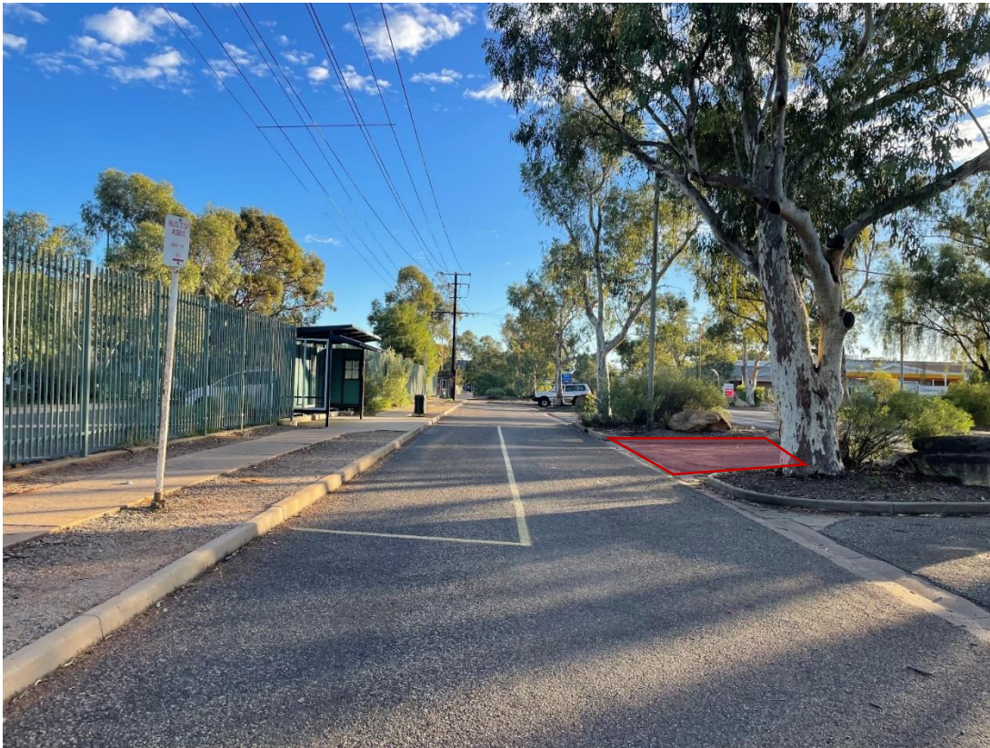
Figure A 6 Faded 40km/h speed limit pavement marking
