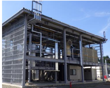
Test facility within Koshijihara Plant (a NEDO* project)
