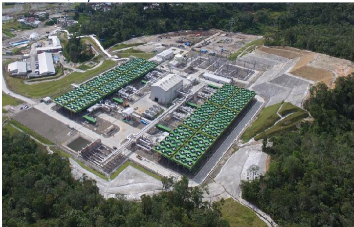
Sarulla Geothermal Independent Power Producer (IPP) Project
