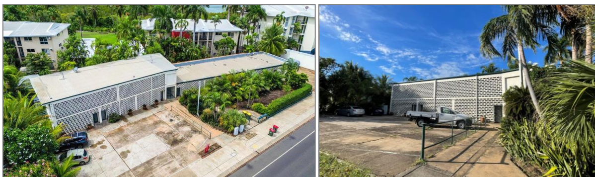
Figure 2: Existing Site Photos
