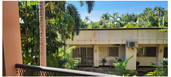
Photo 5: Outlook over single-storey western part of existing complex, as seen from first storey west most block of 73 Progress drive (looking north)
