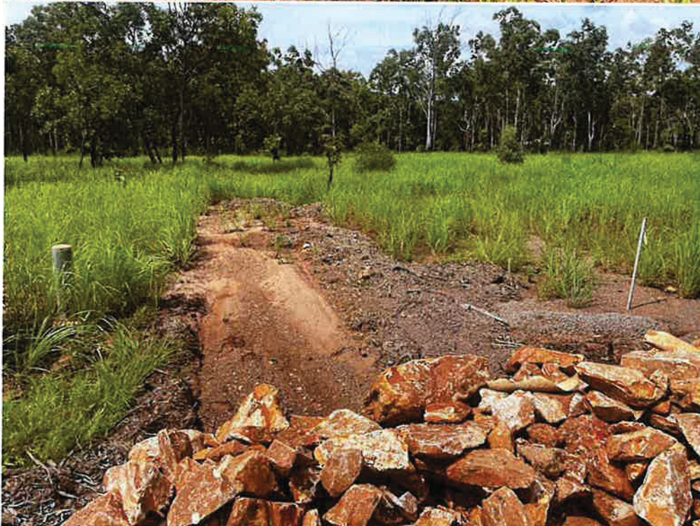
Evidence of Sediment Deposition past breached sections of mulch berm. Sediment to be cleaned up so far as reasonably practicable.
