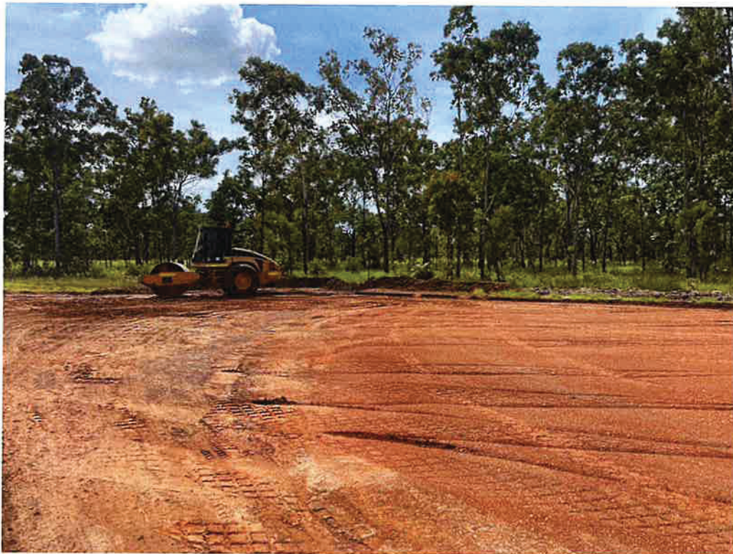
Start of Mulch Berm approx. CH 200. Flows are concentrating and dump rock has been installed where previous breach has occurred. Install Rock Filter Dam.
