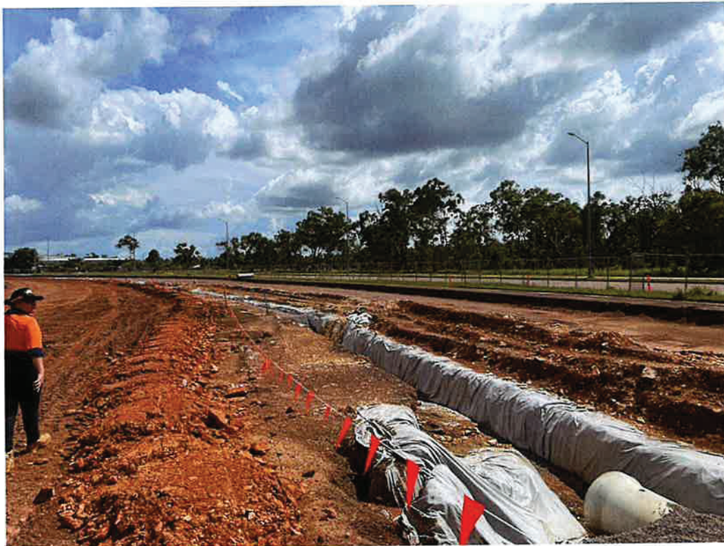
Windrows formed along trench to prevent dirty water ingress
