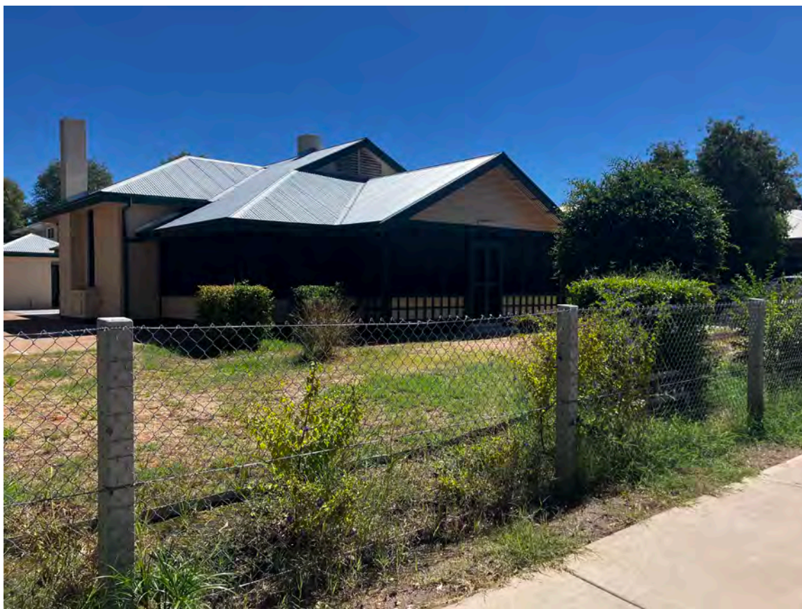
Figure 18 80 Hartley Street, showing completed reinstatement works, Site visit - Planning Officer, captured 2 April 2026.
