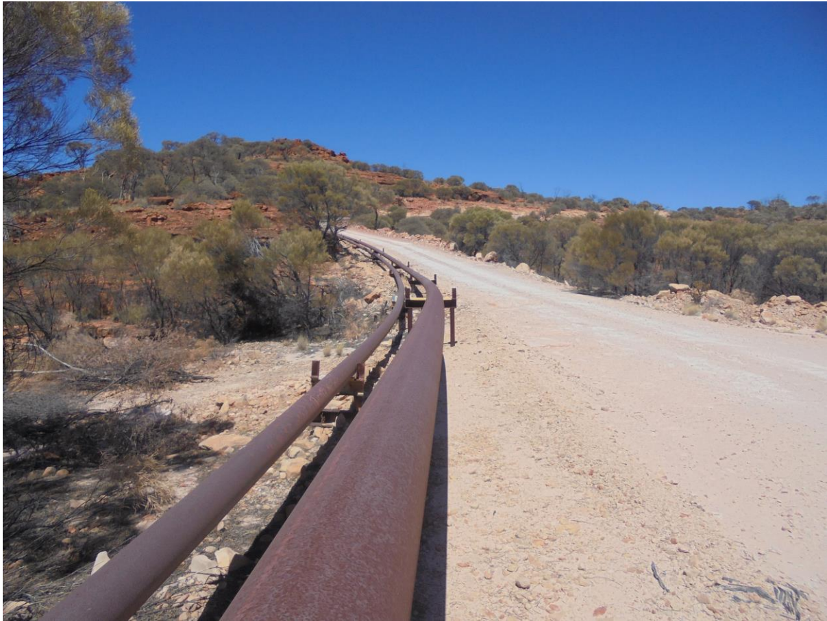
Figure 6-2 Example of a completed flowline and associated pipe stands at the PVGF
