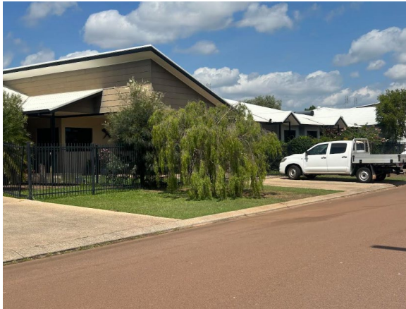
Figure 6 Closer view of duplex on LMR zone
