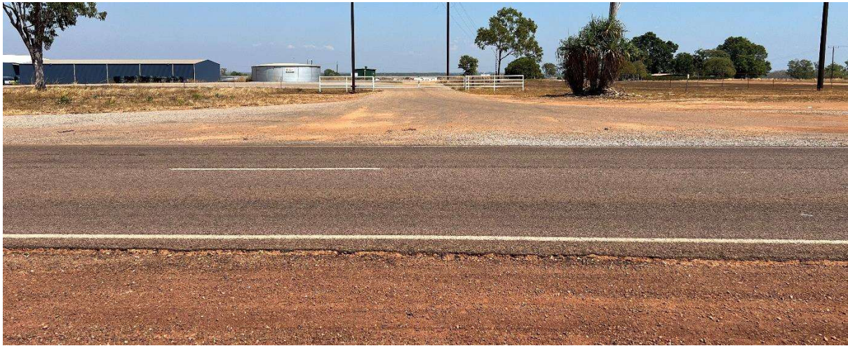
The existing access off the Stuart Highway
