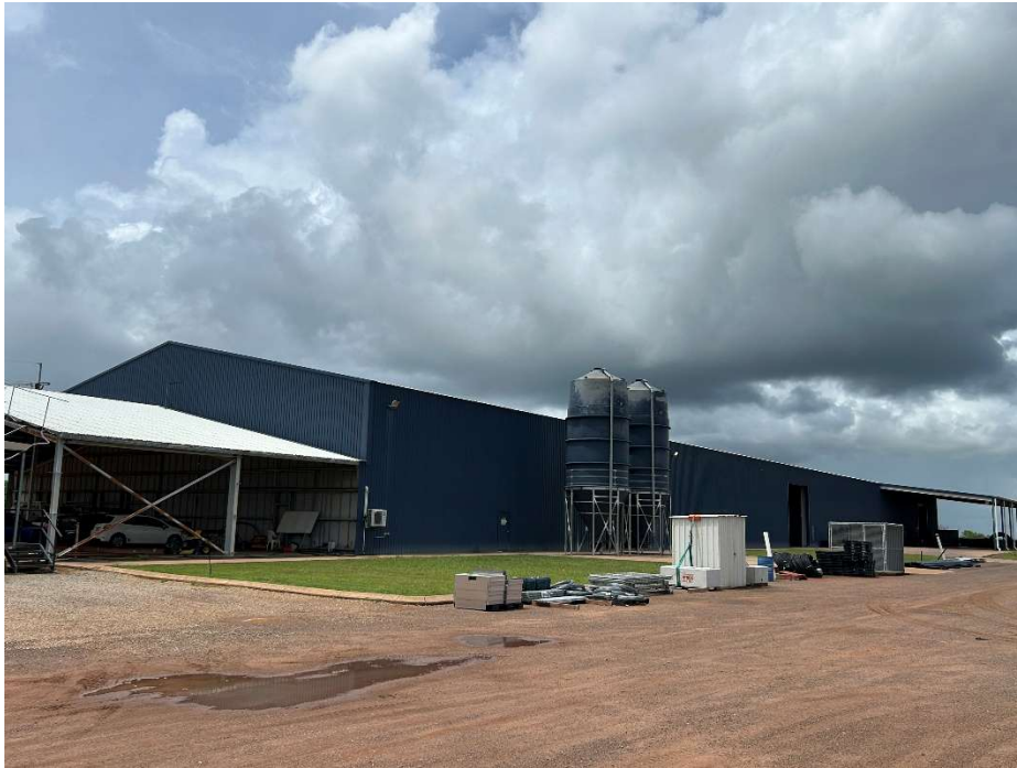
Part of the existing Bilba manufacturing plant
