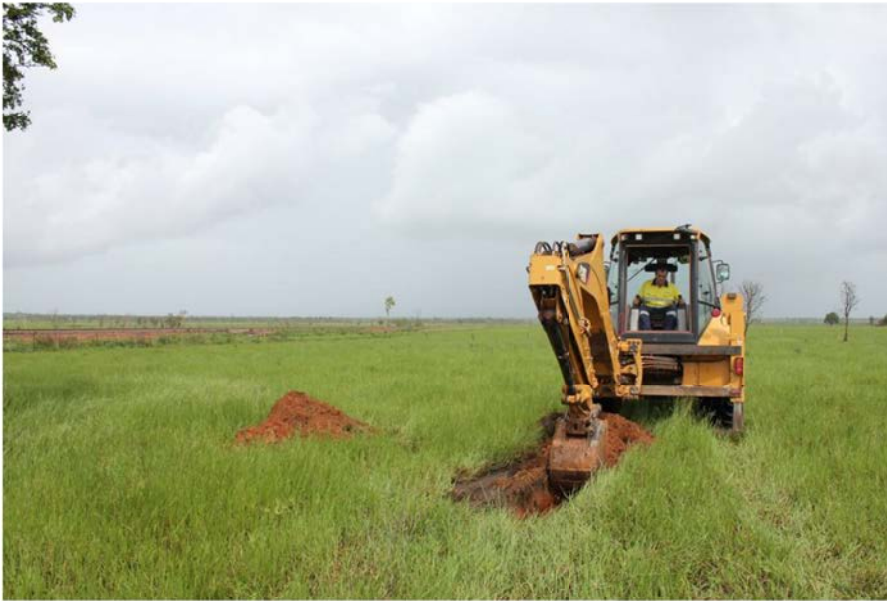
Figure 1 Excavation of Test Pits
