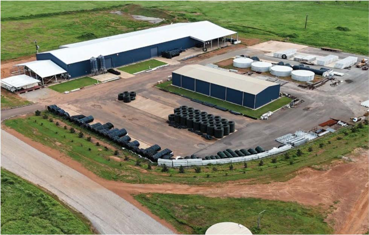
An aerial view of the existing Bilba facility
