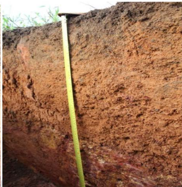
Figure 6 Test Pit 2 Ferricrete (Iron precipitate formed Laterite) is visible at depths below 600mm
