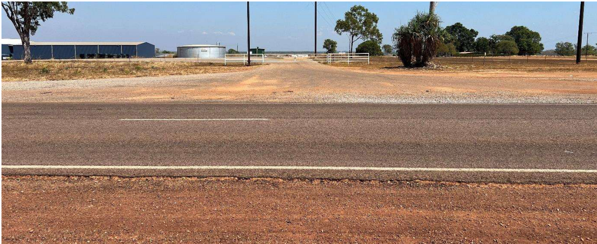
The existing access off the Stuart Highway
