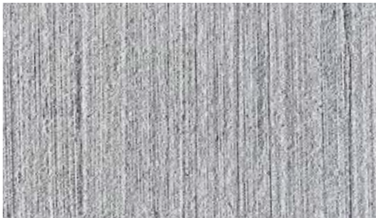
Continous Broom Finish to Concrete (to match Stage One)
