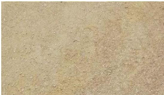
Compacted Rubble pathways
