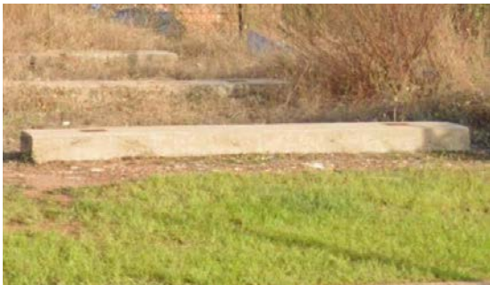
Pre-cast Concrete Footings - Existing reused
