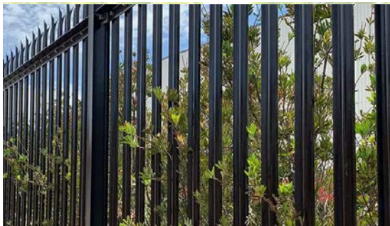
Black Palisade Security Fencing
