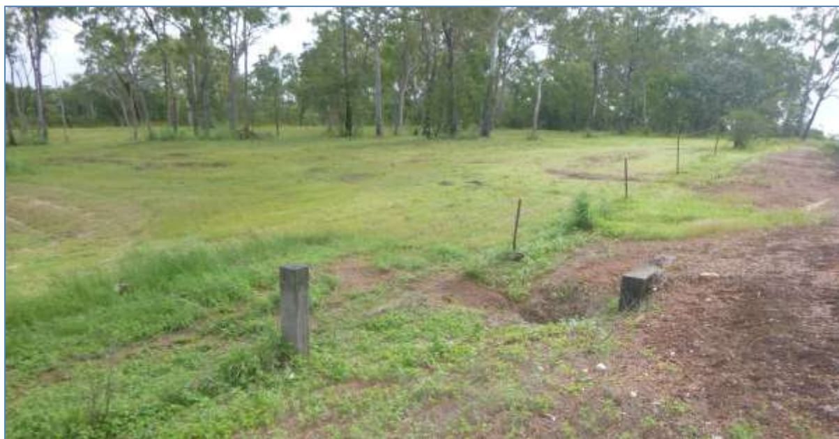
Figure 3 Stormwater drain outlet under Lowther Road discharging into Lot A
