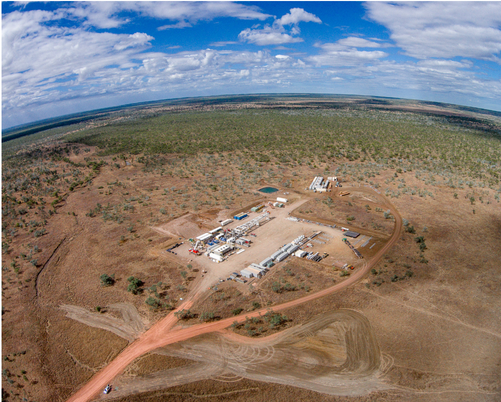
Figure 8: Example of drill rig for site works
