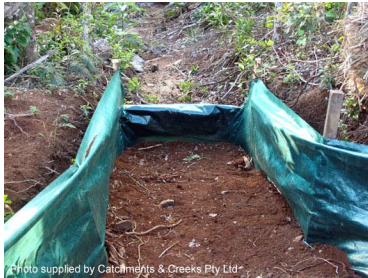
Photo 3 – Up-slope ends of the fence are flared out to adequately capture the inflow
